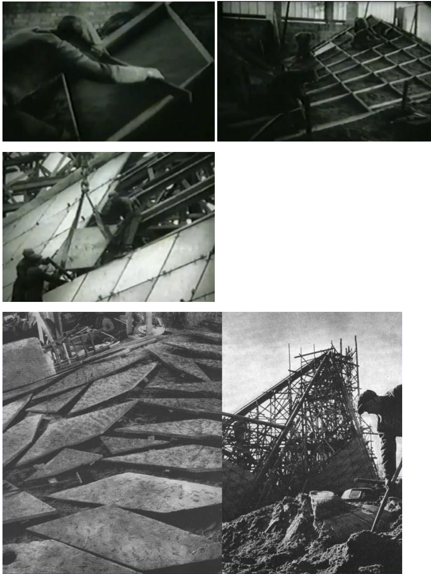
Figures 2.1.3.1a-e Philips pavilion under construction.
