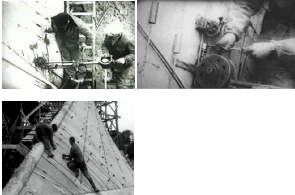
Figures 2.1.3.2 a-c Philips Pavilion under construction
