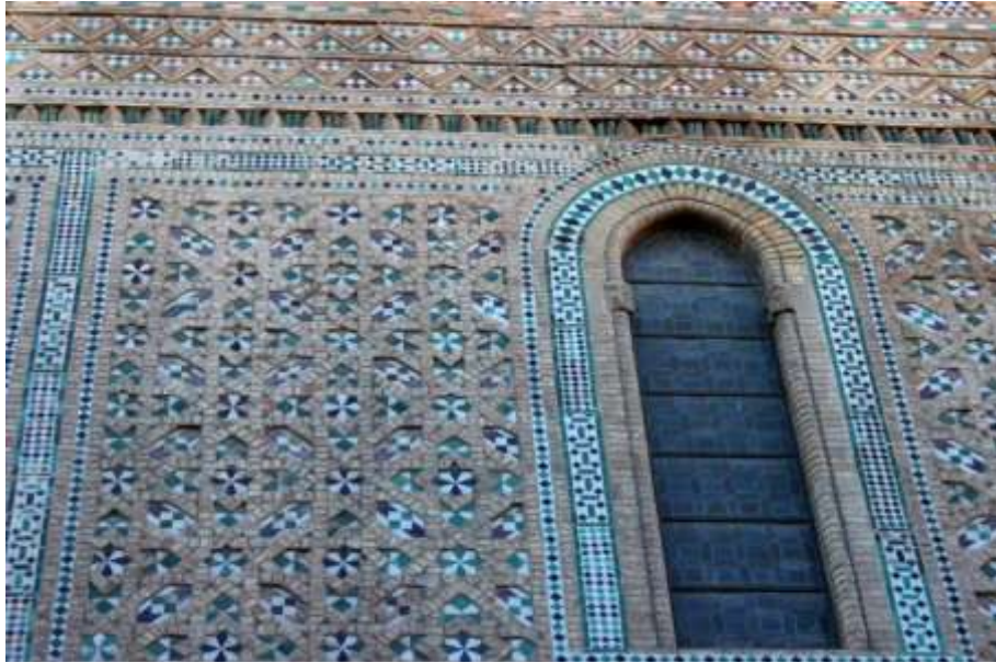
Figure 107. The Cathedral Seo, Mudéjar brick and ceramic details, Zaragoza (taken by the author)
