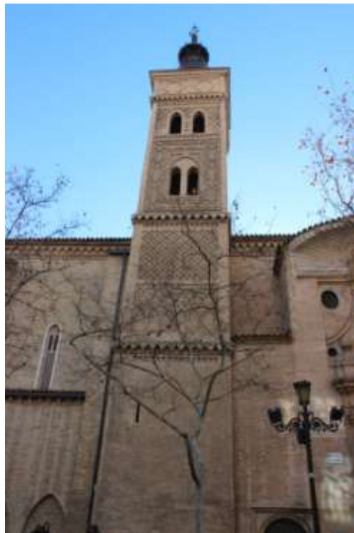
Figure 111. The Church of San Miguel de los Navarros, 14th century, Zaragoza (taken by the author)
