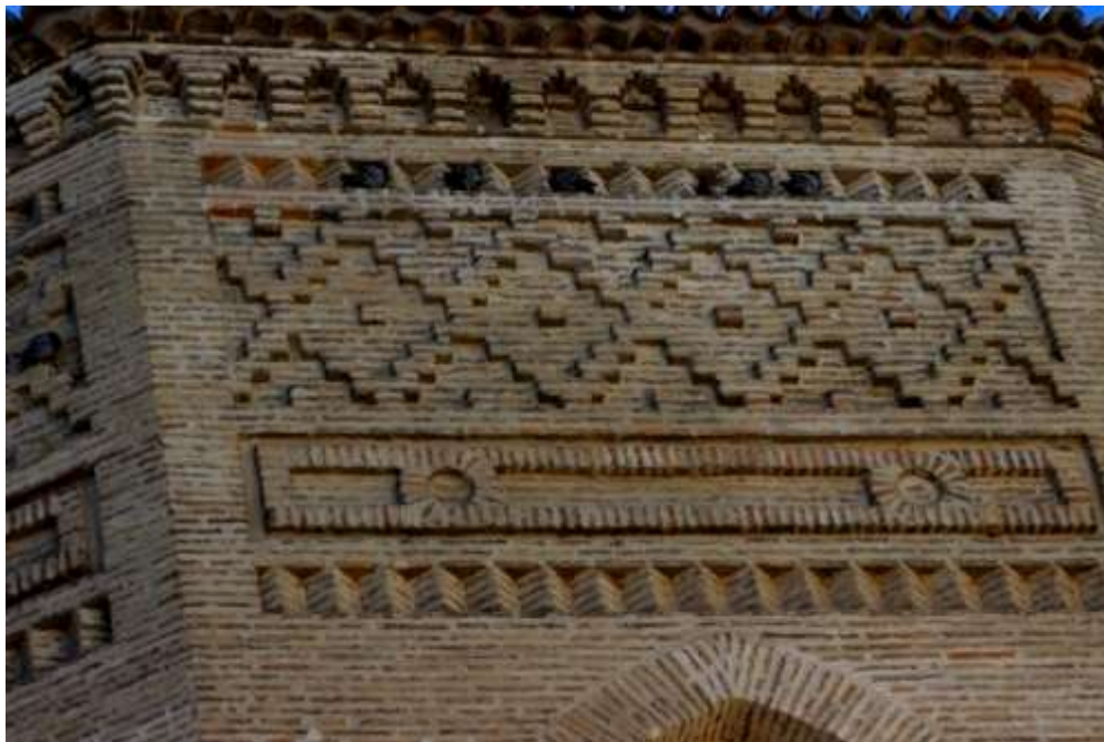
Figure 49. Brick as a construction and decoration material, the Santa Maria Magdalena Church, 14th century, Zaragoza (taken by the author)
