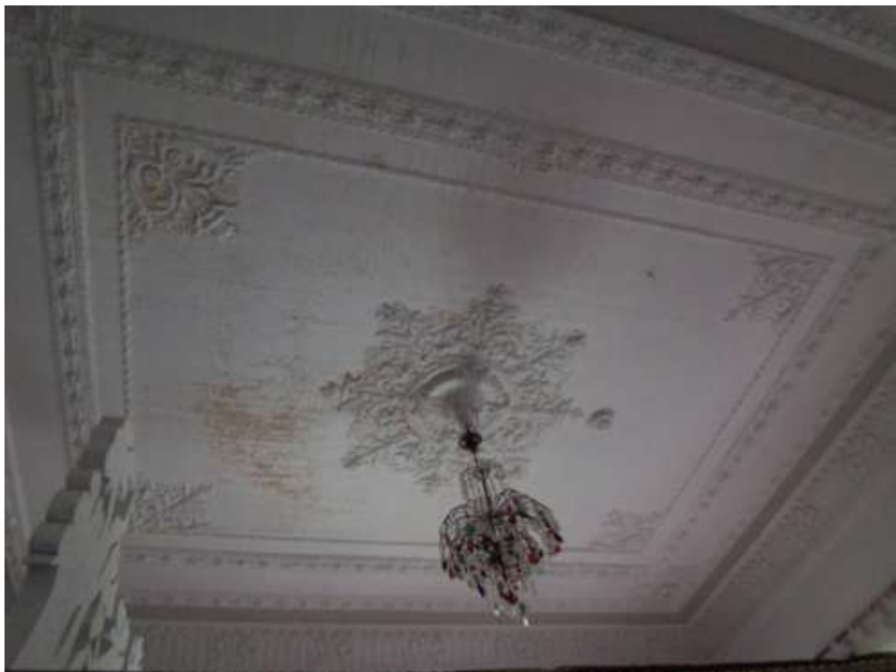
Photo 4.3.69 The ceiling of the room on the front-right
