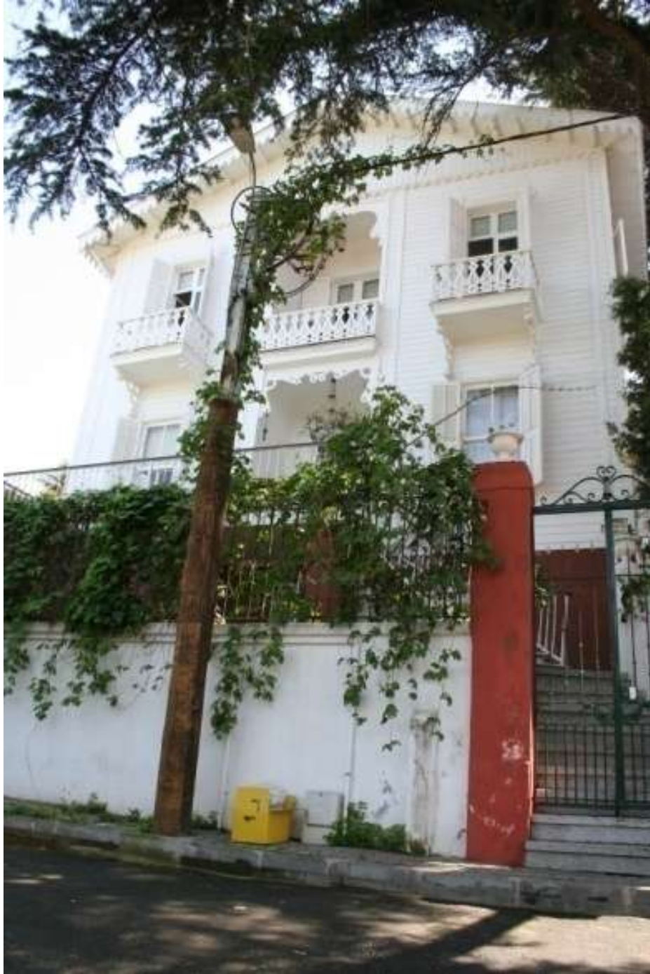
Photo 4.3.38 The front view from Peltek street
