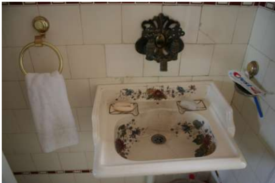
Photo 4.3.28 The original wash basin
