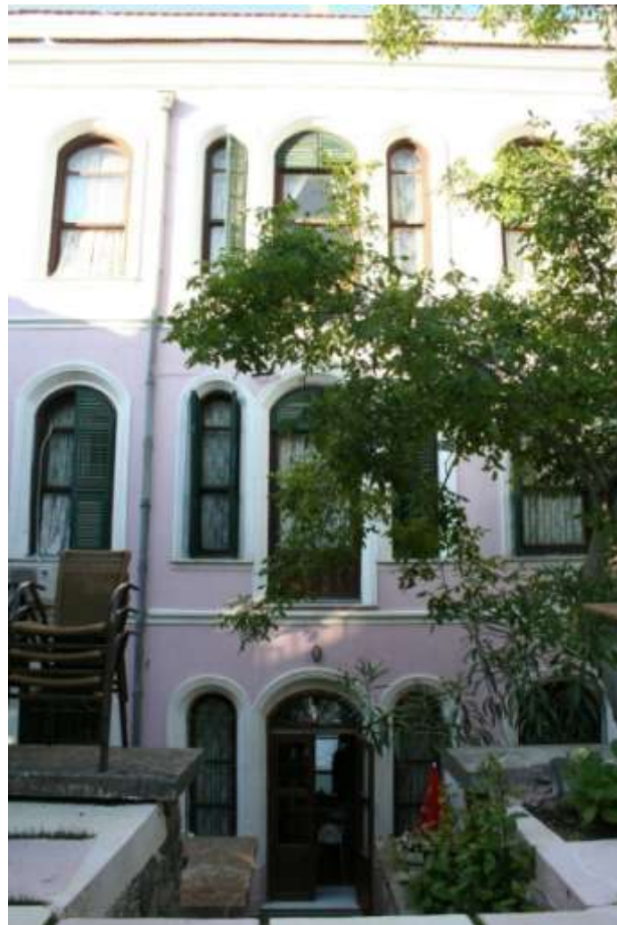
Photo 4.3.120 The back view of Meziki Mansion
