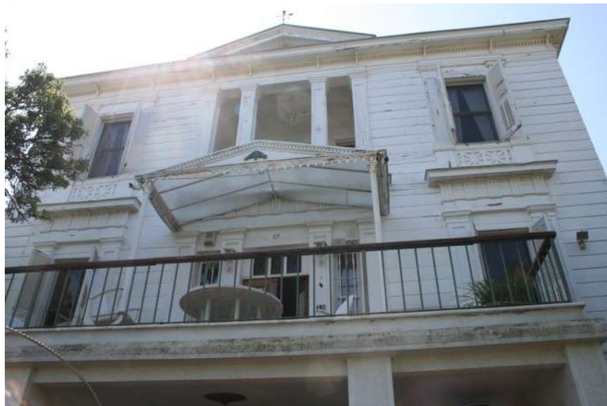
Photo 4.3.21 Front view looking below the entrance terrace
