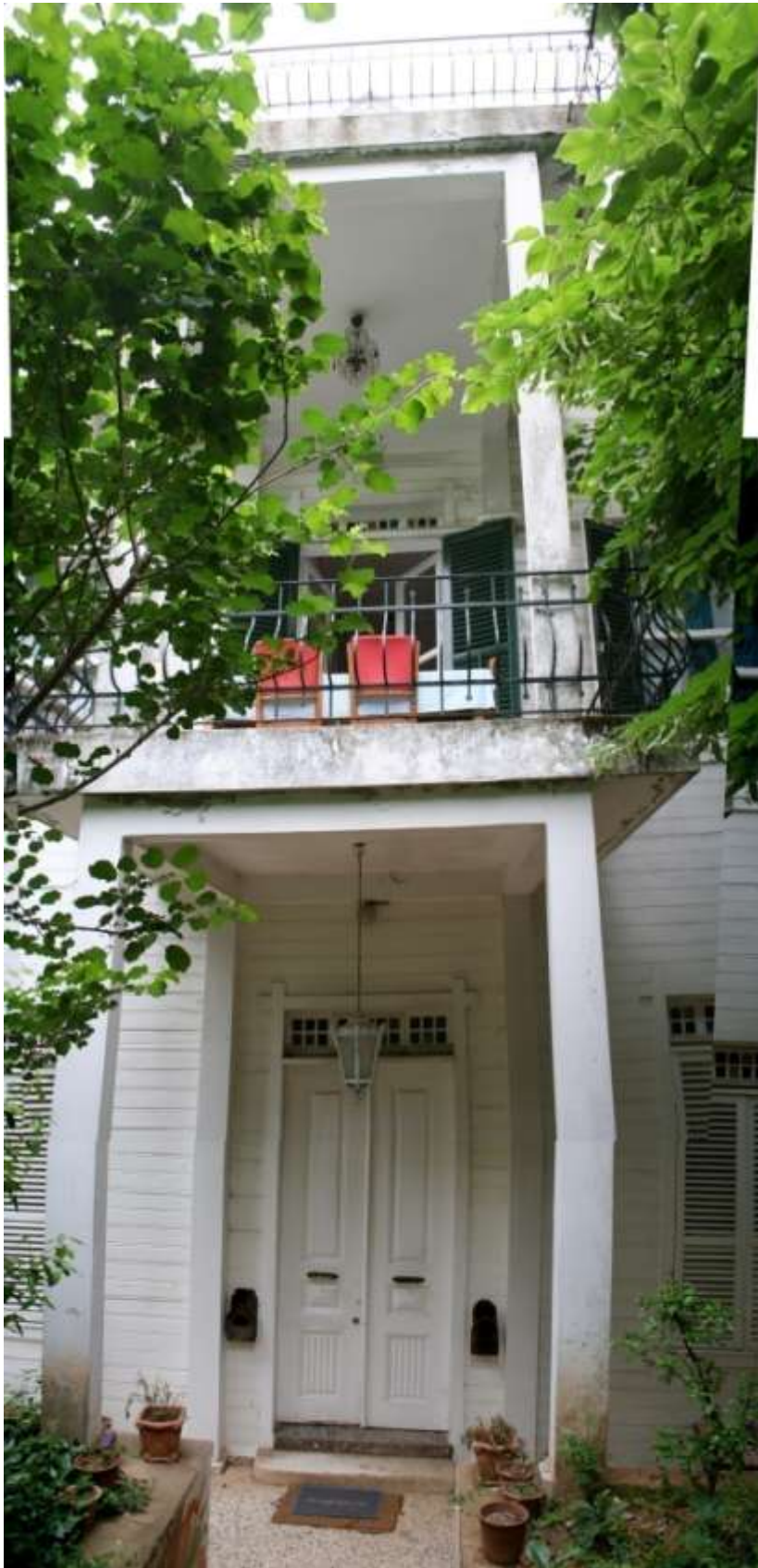
Photo 4.3.63 The back view
