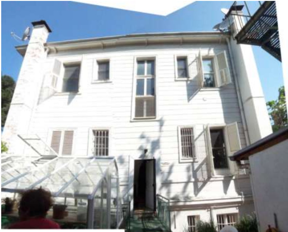
Photo 4.3.36 Back view of Farra Mansion
