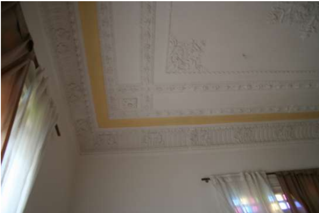
Photo 4.3.67 Ceiling detail from the front-right room
