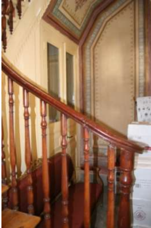
Photo 4.3.111 Detail from the staircase, see the doors opening to merdivenaltı which is used as storage
