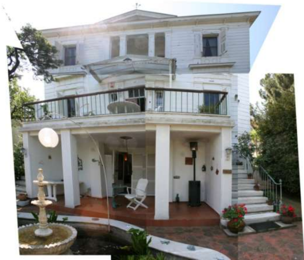
Photo 4.3.20 Collage showing the front view of Farra Mansion
