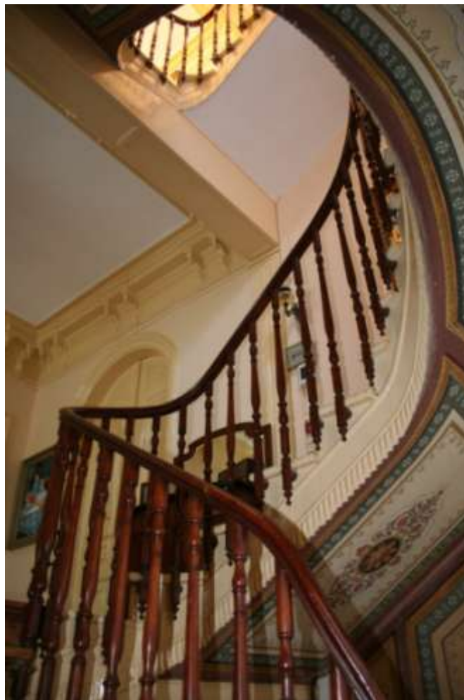
Photo 4.3.118 Climbing up the stairs
