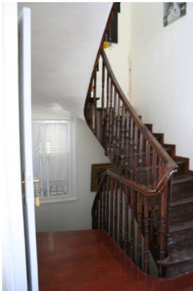
Photo 4.3.46 The wooden staircase
