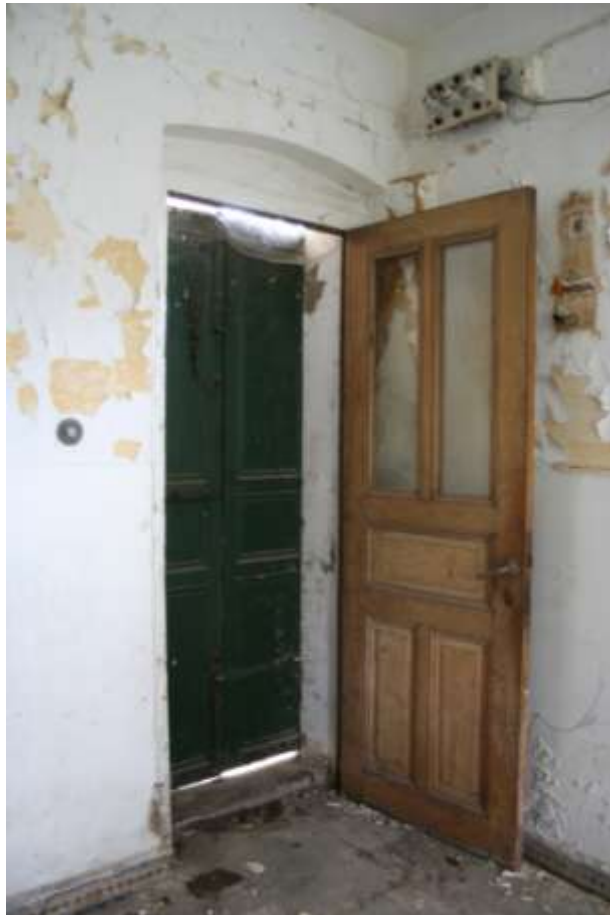
Photo 4.3.101 The door, opening to the garden from the kitchen
