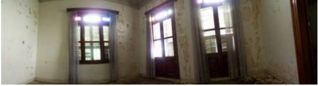
Photo 4.3.91 The reception room of the grandmother on the front-left side
