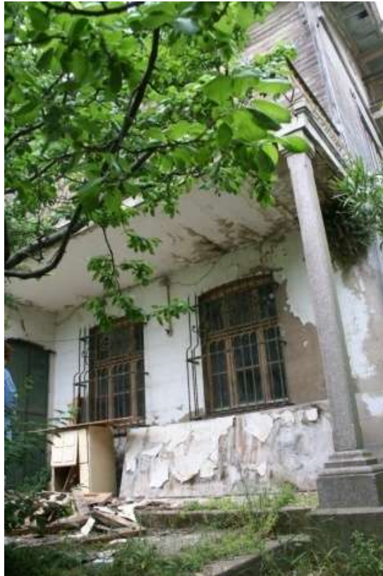
Photo 4.3.86 The front view of Usulcuoğlu Mansion
