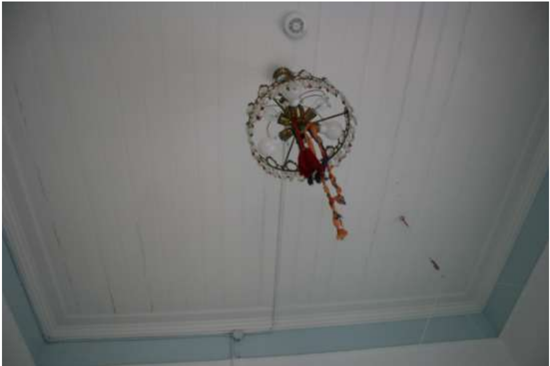
Photo 4.3.75 The ceilings of the back rooms are without ornamentation
