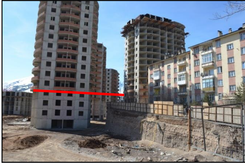
Figure 23. The storeys below the red line did not included in the calculation of floor area ratio.
