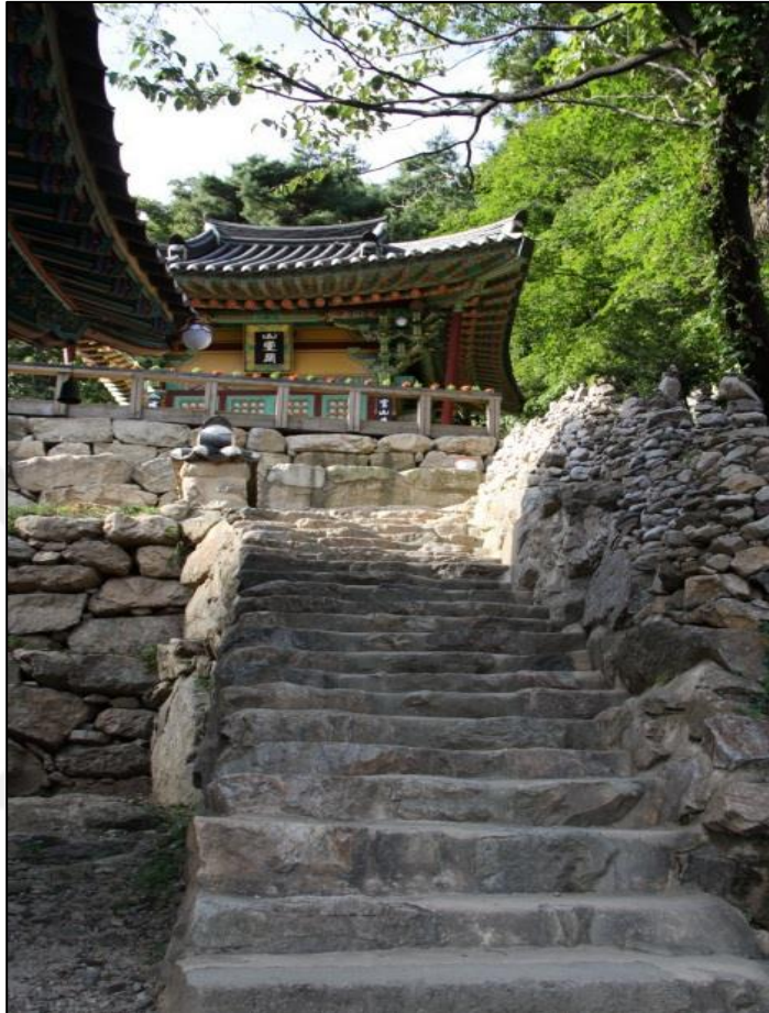
Figure 105 Stairs of Youngmunsa Temple in Yang Pyeong
