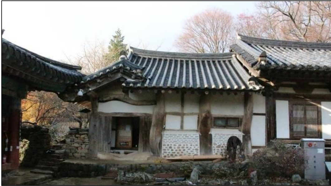
Figure 116 Natural Wodden Beams and Columns are Used in Gesimsa Temple, Built in 14 th Century by Chungsook
