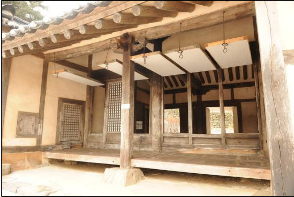
Figure 68 No Distinction Between Windows and Doors in Asan Mang's Residence, Built in 14 th Century
