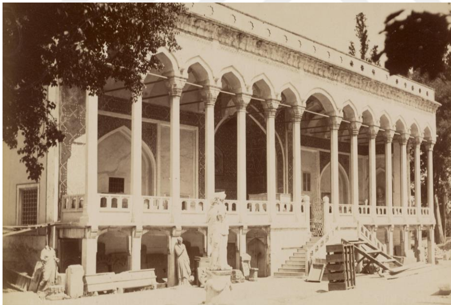
Figure 4 The Tiled Kiosk after renovation
