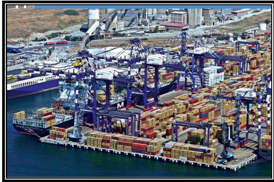
Figure 3.6. General View of MARPORT Main Terminal (Source, www.marport.com.tr , 2016).
