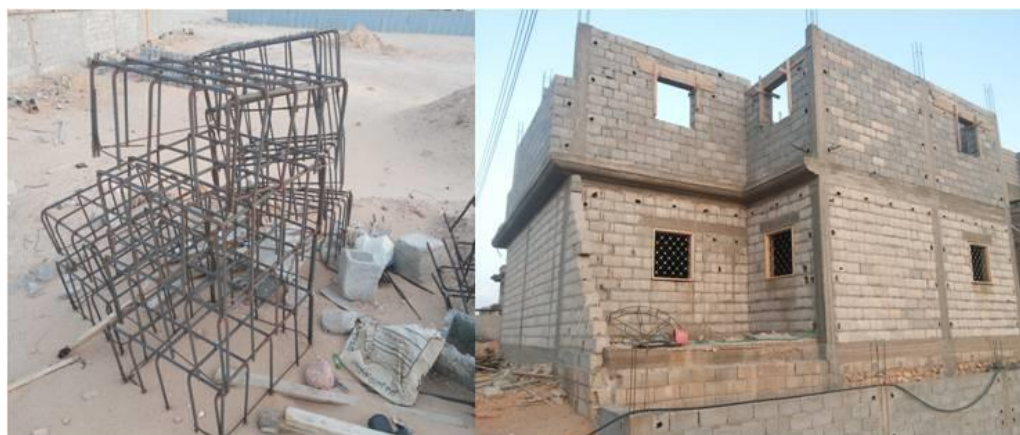
Figure (3.17) Constructional Steel and Hollow Concrete Blocks. By author.
