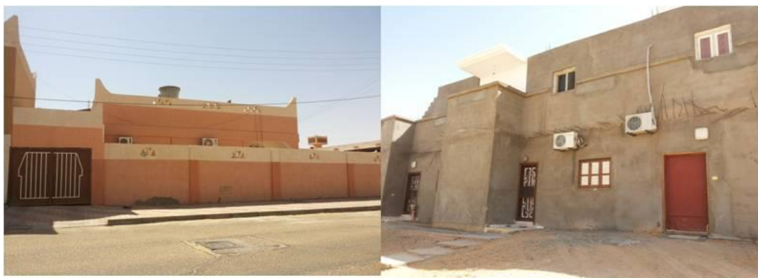
Figure (5.12) Using Electrical Air Conditioner in Contemporary Houses.
