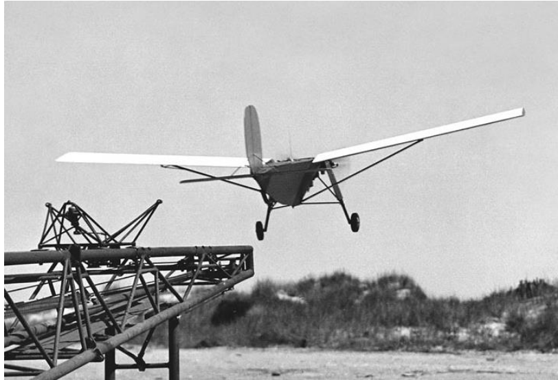
Figure 1.8 A Radioplane OQ-2 and its launcher [10]
