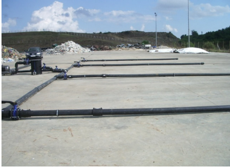
Figure 3.2 : Aeration system used in aerated static pile.
