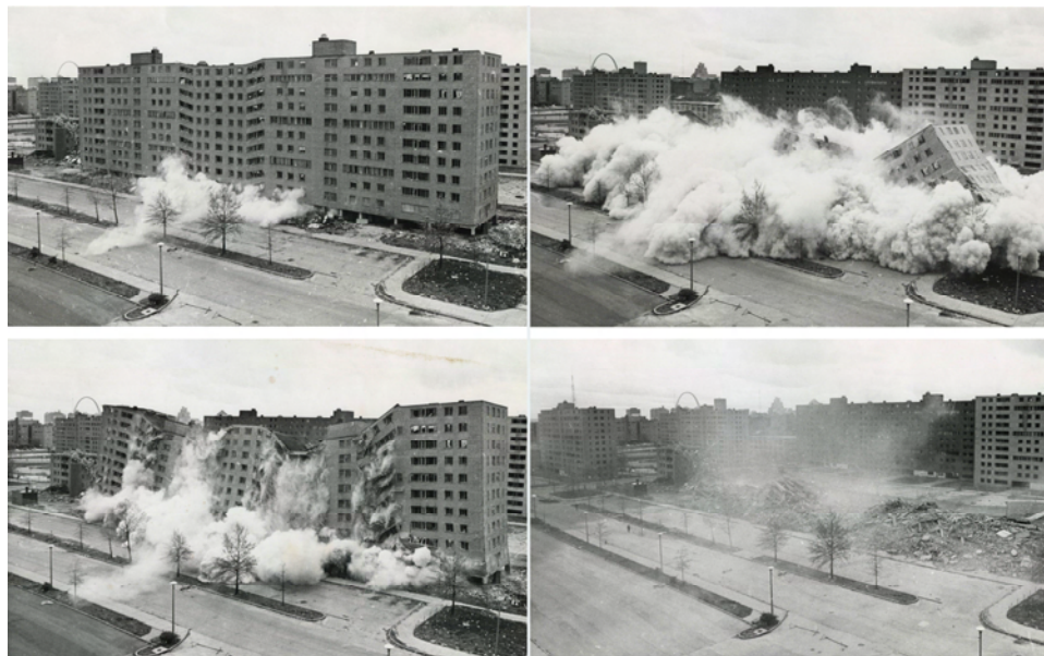
Figure 1.1 : Demolition of Pruitt Igoe-1972, (Url-2)
