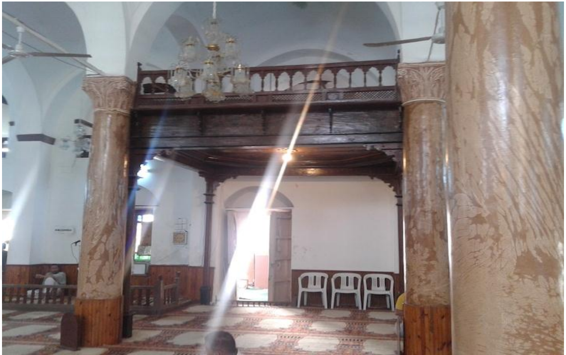
Figure 17: The first floor of Shayib Aleayn Mosque
