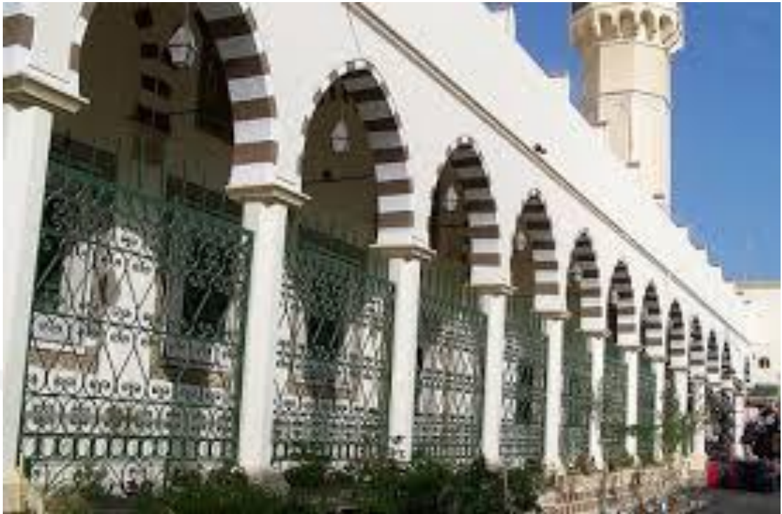
Figure 5: The external interface of Ahmed Pasha Mosque
