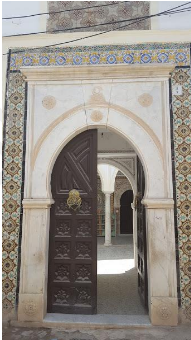
Figure 3. 64: The Eastern Exterior to the Prayer Hall in Mustafa Gurji Mosque (Source: by the researcher)
