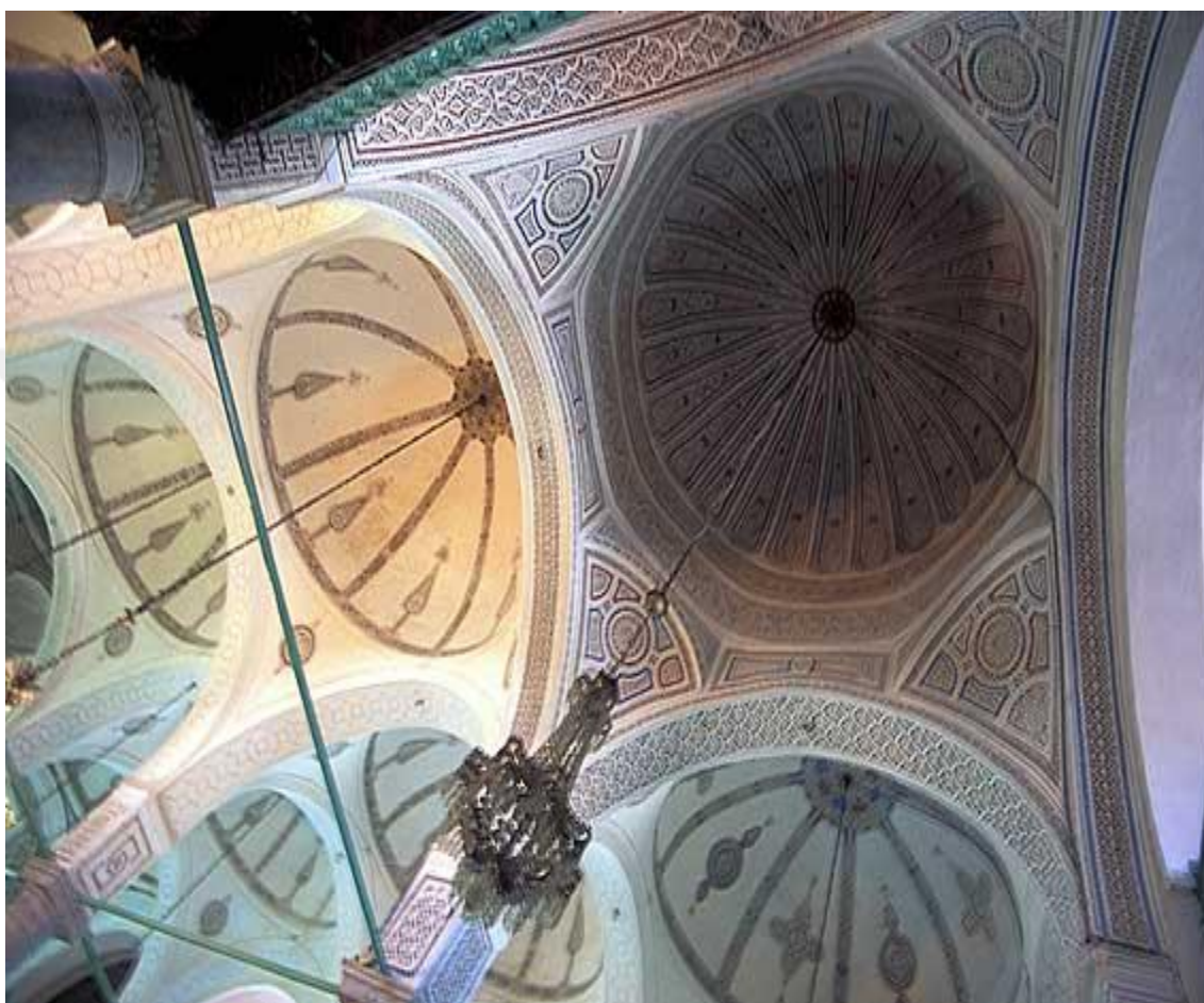
Figure 3. 77: A General Picture of the Roof of the Mosque Showing Domes
