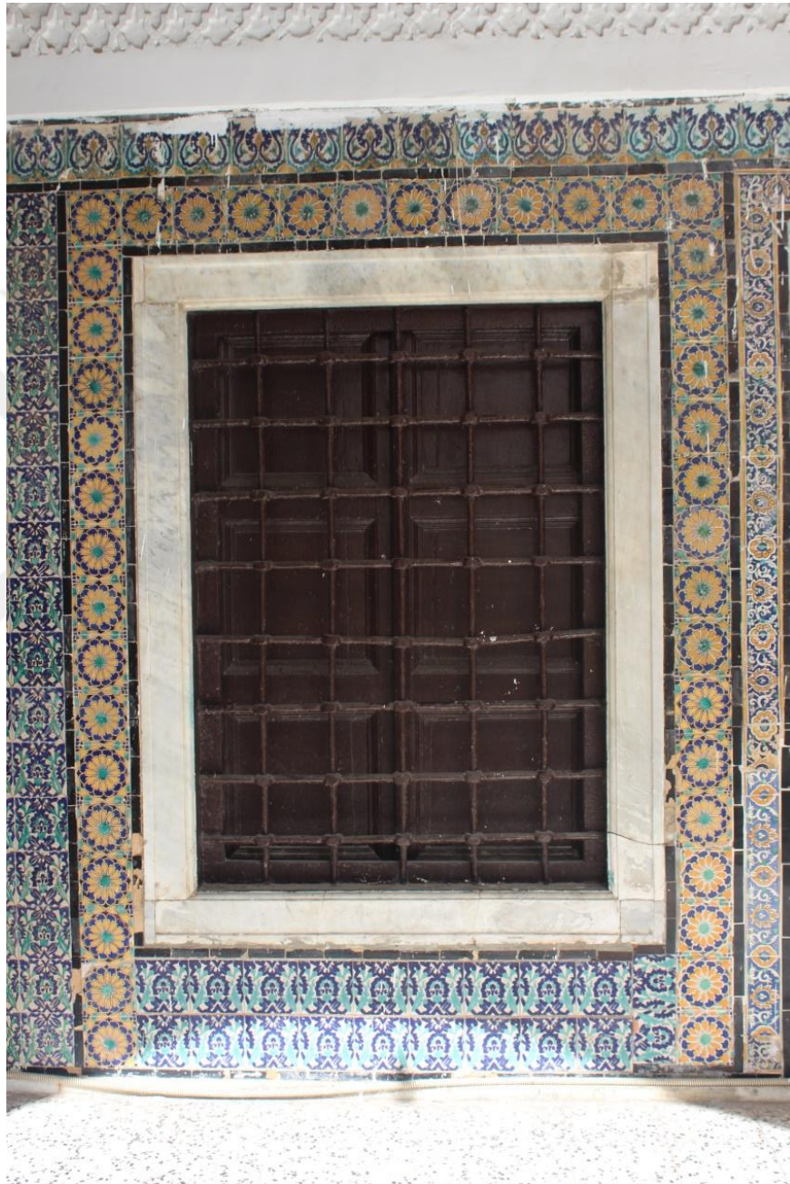
Figure 3. 47: General Picture of the Decoration the Ceramic Also Shows The Windows
