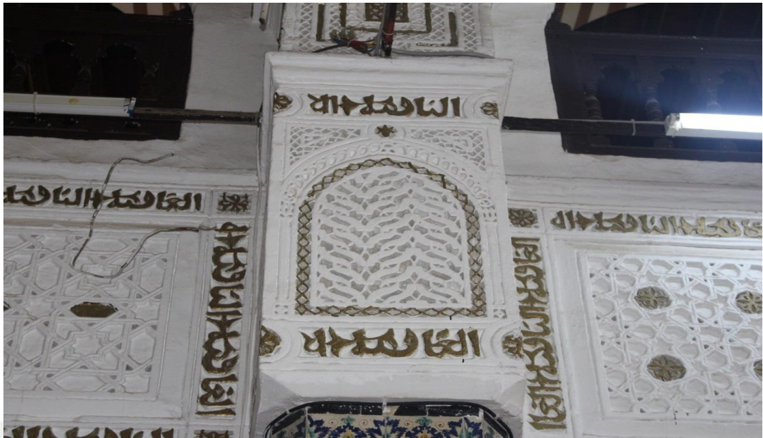
Figure 3. 55: A Gypsum Board in Ahmed Al-Qaramanli Mosque (Source: by the researcher)
