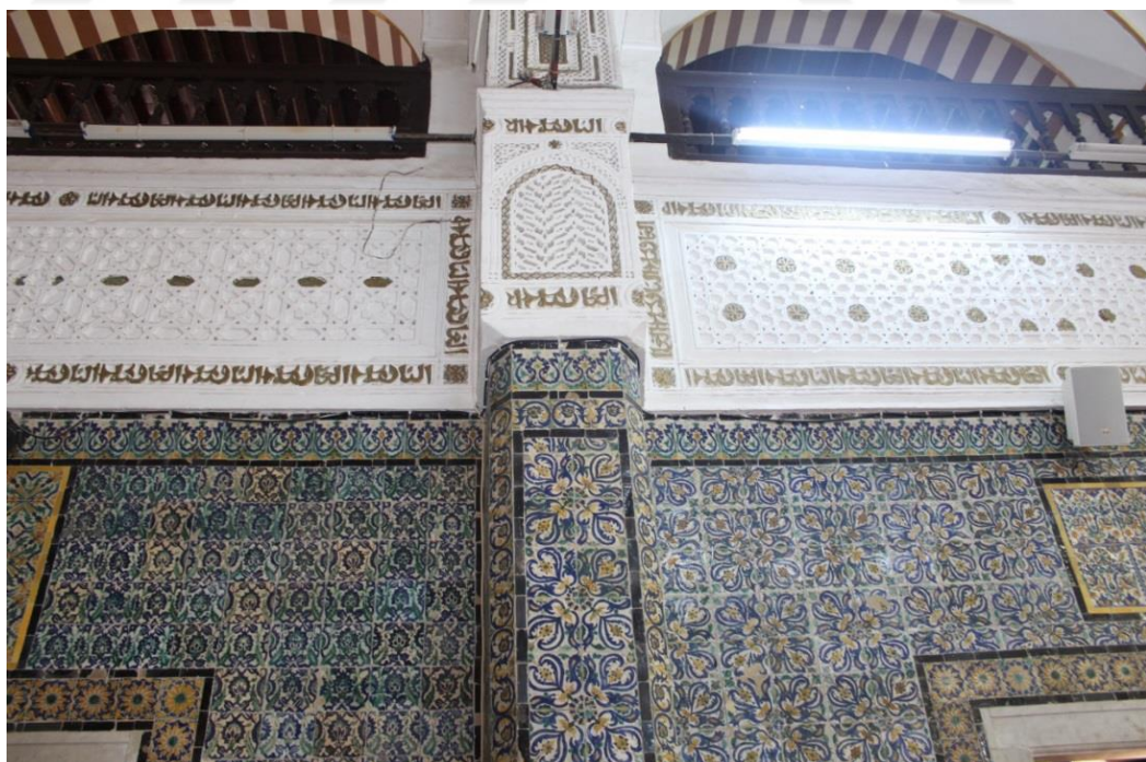
Figure 3. 54: A Gypsum Board in Ahmed Al-Qaramanli Mosque (Source: by the researcher)
