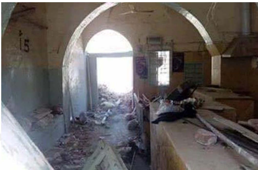
Figure 3. 19: A Photograph Showing the Demolition of the Historic Al Adlouni Hotel
