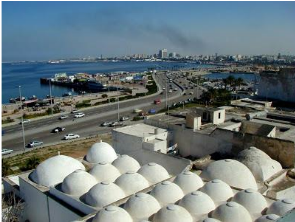
Pic.(12) New picture shows the Domes of Darghut Pasha Mosque
