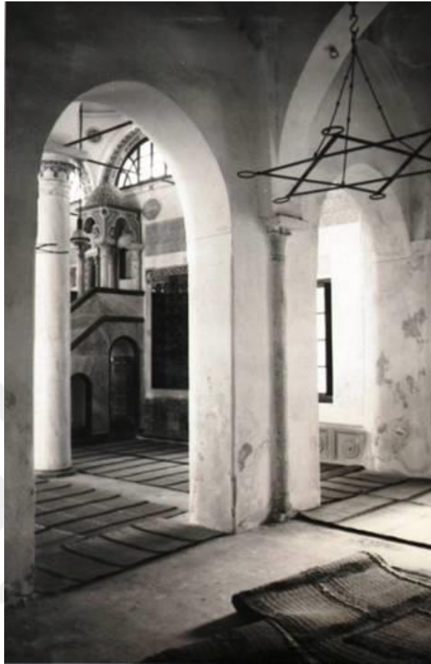
Figure (A) House of prayer and part of rostrum Darghut Basha Mosque
