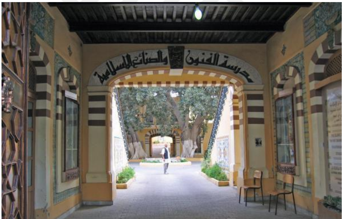
Figure (M). The main entrance of the Islamic Arts and Crafts School
