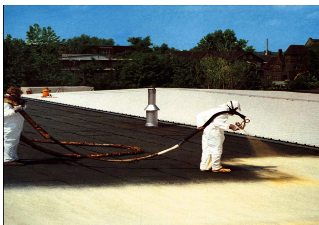
Figure 2.8 : Thermal insulation and sealing in one operation [13]
