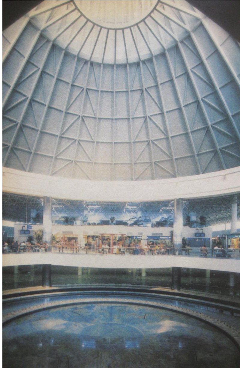
Figure 3.25: Antalya Airport International Lines Terminal Building I, Tekeli-Sisa Antalya, 1991-1998, the first prize in the competition with limited participation held by Directorate General of State Airports Administration (DHMI). (Ekincioglu, 2001c).
