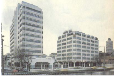
Figure 3.69 : Bank and office building complex, Tekeli-Sisa, Istanbul, 1976-1999. (Ekincioglu, 2001c).
