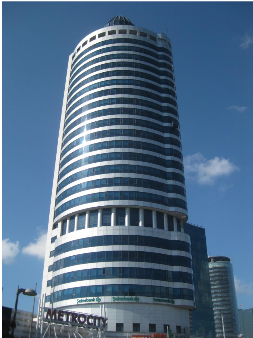
Figure 3.107 : Metrocity Shopping, Office and Residence Complex, the office block. (Photograph: Meral Ekincioğlu).
