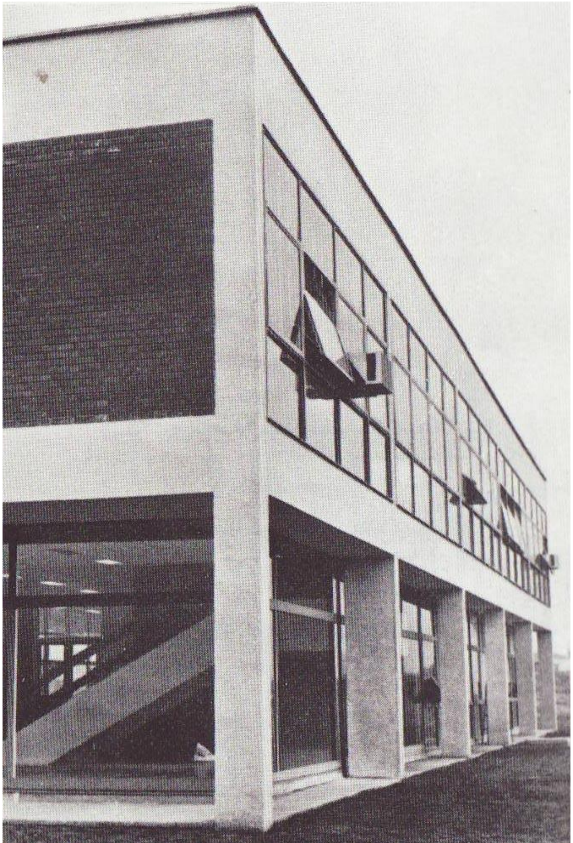
Figure 3.53 : Chrysler Truck Assembly Plant, administrative block. (Tekeli and Sisa, 1976).
