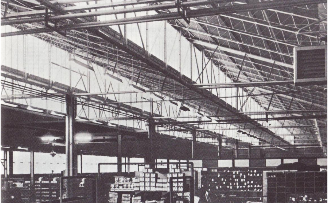
Figure 3.50 : Chrysler Truck Assembly Plant, interior. (Tekeli and Sisa, 1976).
