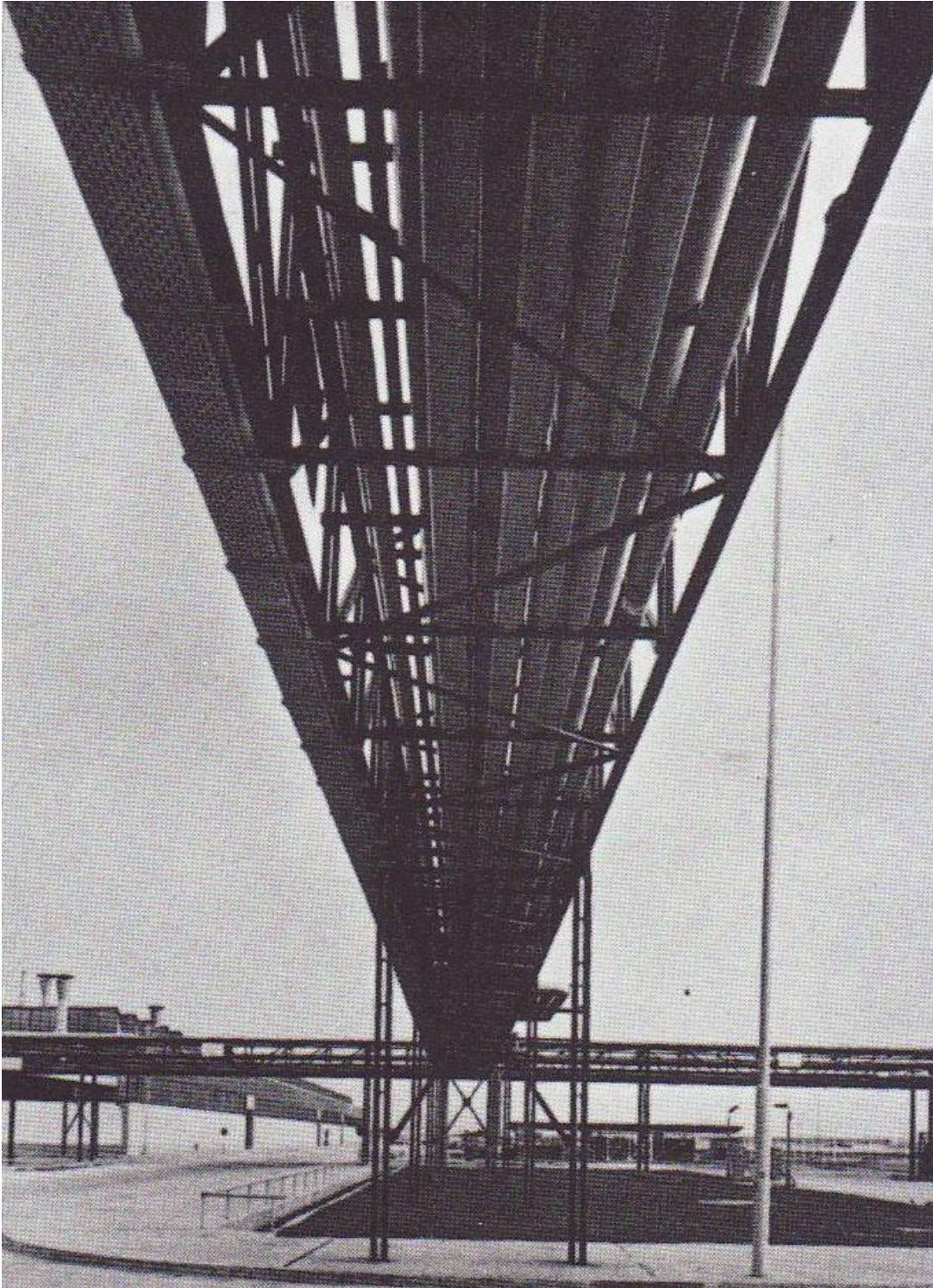
Figure 1.7 : Renault Car Manufacturing Plant, Tekeli-Sisa, Bursa, 1971-1972, bridges ensuring utility distribution from the boiler room to all buildings. (Tekeli and Sisa, 1976).
