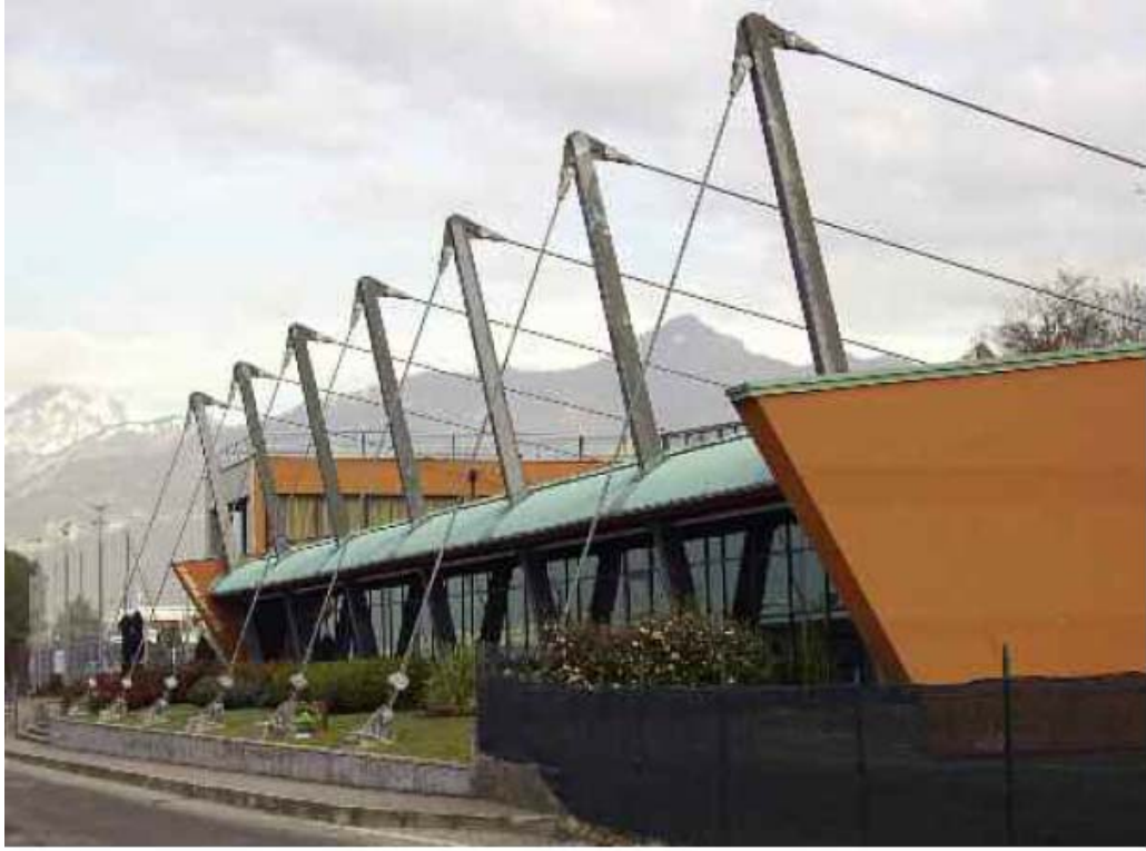
Cable stayed roof, 26 m span.
