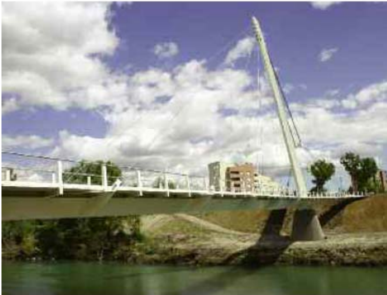
Stayed footbridge with sloping mast, 74 m span. Stay cables FLC 54 and FLC 32.
