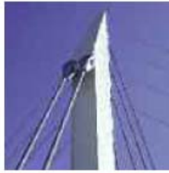
Cable stayed footbridge, 43 m span. Stay cables OSS 17 and FLC 55, 86.
