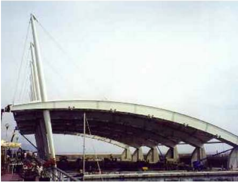
Suspension roof steel/membrane system. Suspension cables FLC 30.
