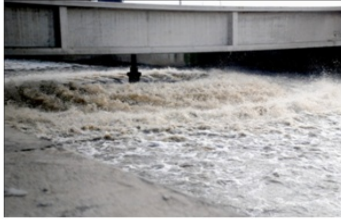
Figure 3. 5: Photograph of mechanical surface aerators.
