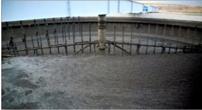
Figure 3. 6: Photograph of primary sludge thickening tank.
