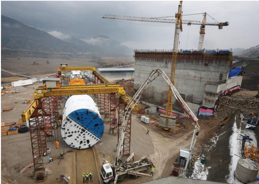
Figure 6.14 : Assembly on the jobsite (Willis, 2012).
