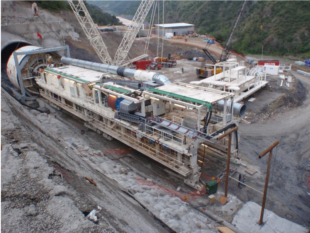
Figure 6.2 : TBM assembly at the portal.
