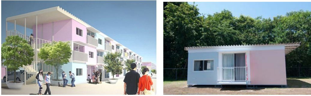
Figure 2.9 : Multistory temporary housing designed by Shigeru Ban after the Japan earthquake and tsunami (Url-6).
