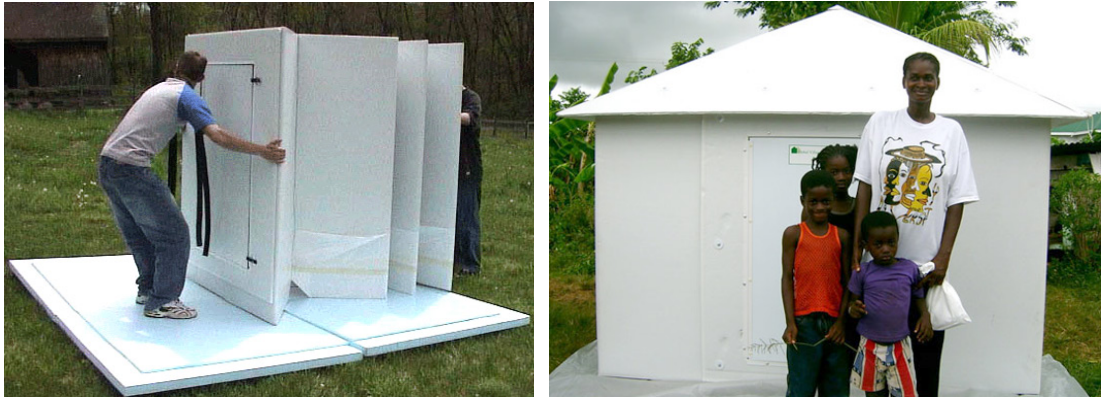
Figure 2.7 : Images demonstrating the installation and usage of the flat pack shelter (Url-4).
