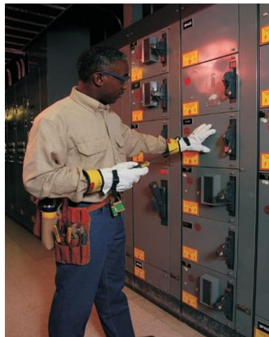
Figure 2.21 : A protective shirt which is made of Polypropanoate(acrylic), Aramid and Polyamide fibers' mixture.
