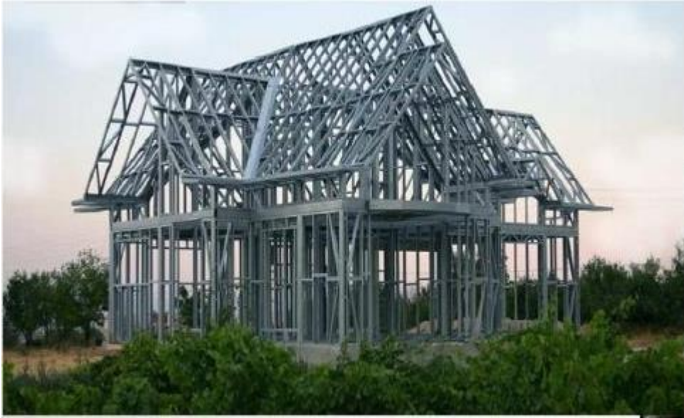
Figure 1.4 : Cold formed steel building example [6].
