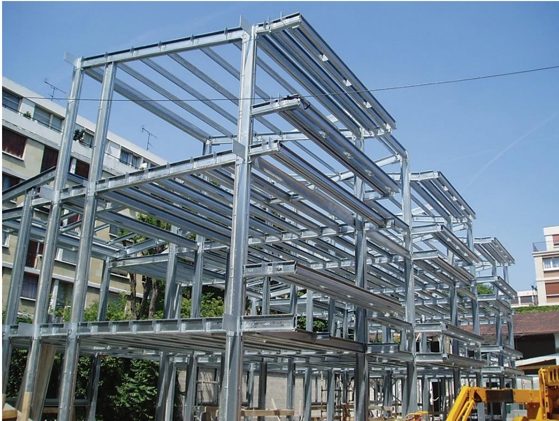
Figure 1.5 : Cold formed steel structure example [7].
