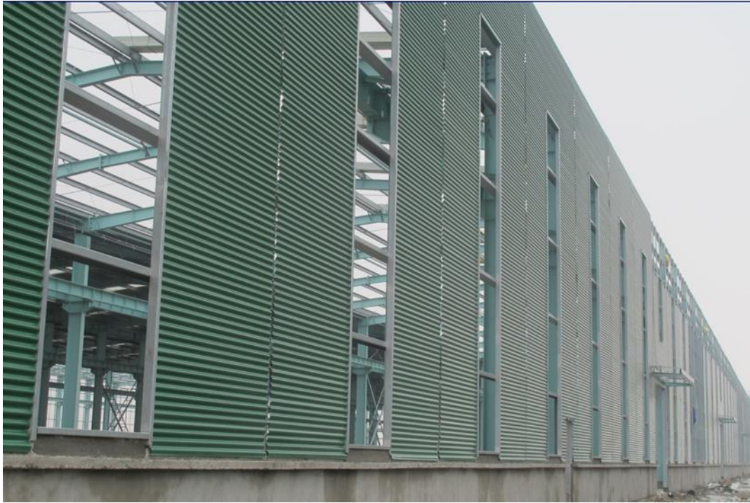
Figure 1.10 : An example of cold formed wall panel [11].
