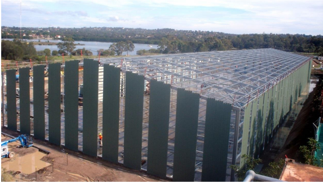
Figure 1.6 : A cold formed steel hangar [8].
