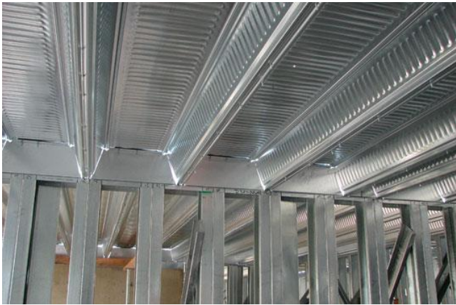
Figure 1.9 : Cold formed steel roof deck example [10].
