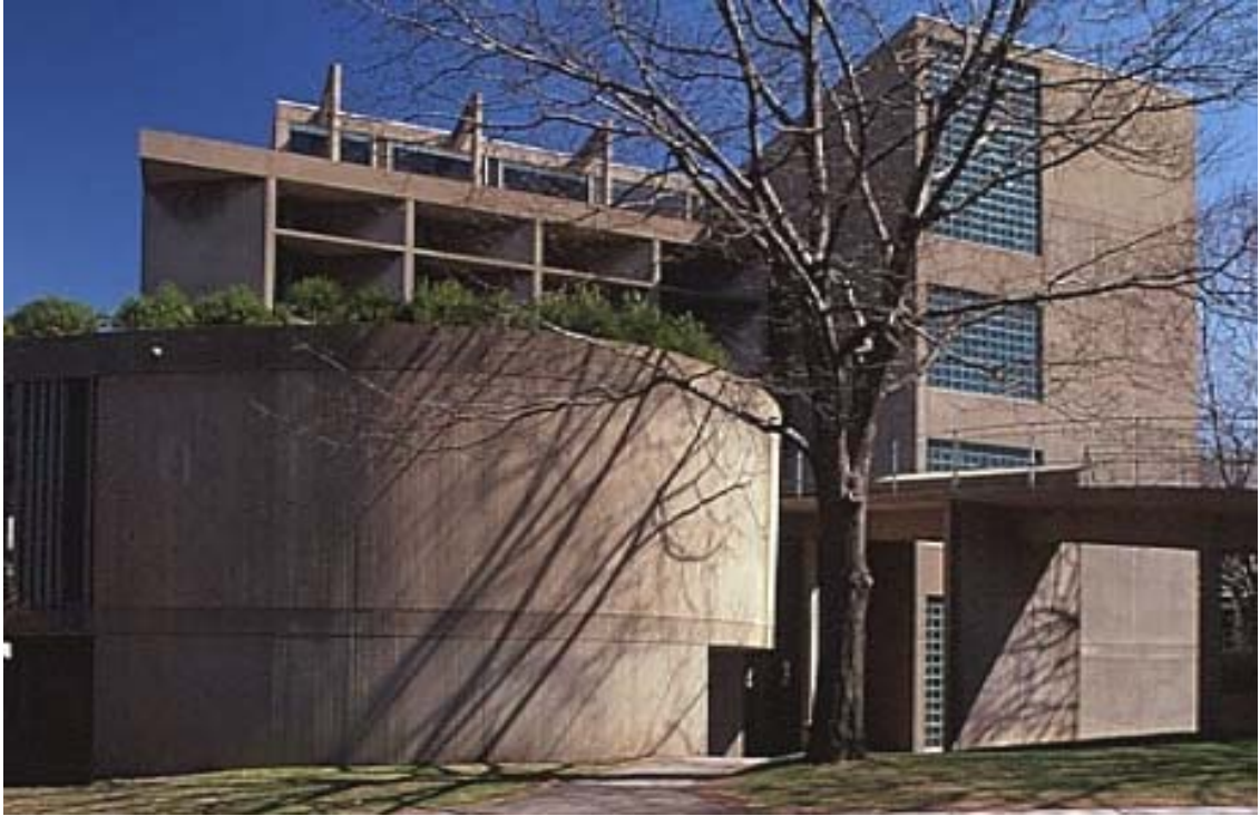
Figure 8. Carpenter Center for the Visual Arts (1961) by Le Corbusier (Source: http://www.worldandi.com/newhome/public/2003/august/arpub.asp )
