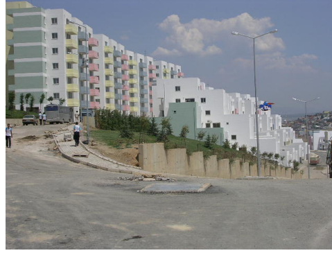
Figure 4.2. View of apartment blocks in Athletes' Village
