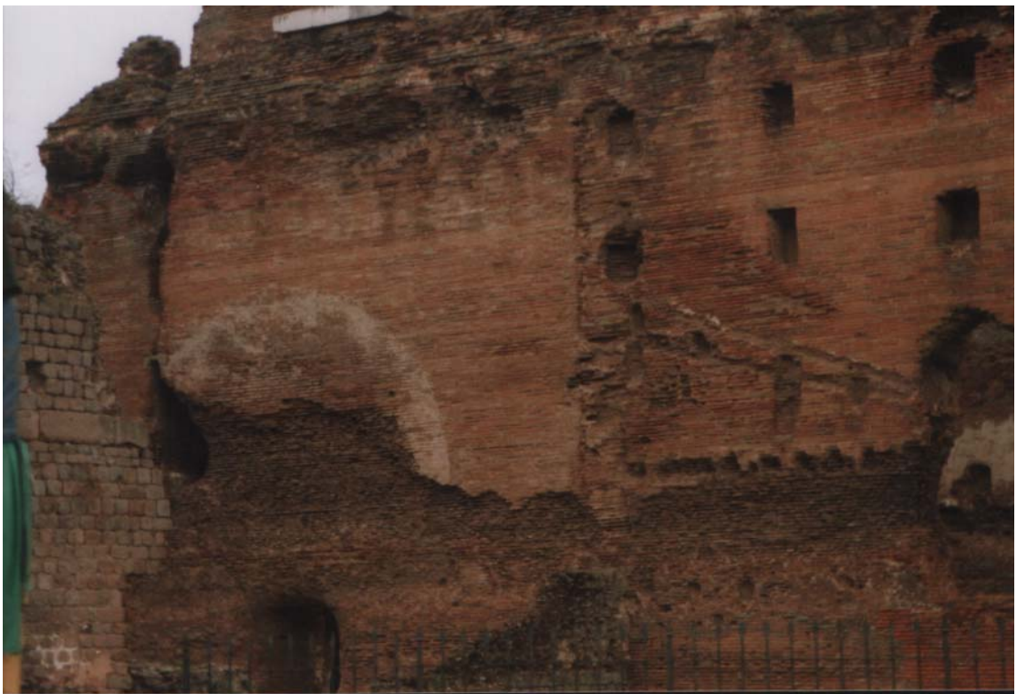
Figure 4. 96. Loss of material in the north-east elevation (2004)
