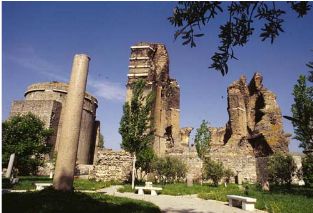
Figure 2. 3. South-east facade of the Serapis Temple (Photograph: Website of Ministry of Konak )
