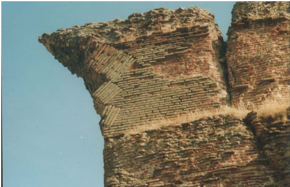
Figure 4. 94. Growing of micro organisms on the brick surfaces (2004)
