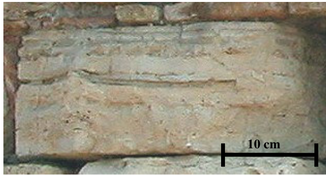
Figure 3.8. Weathering out dependent on stone structure
