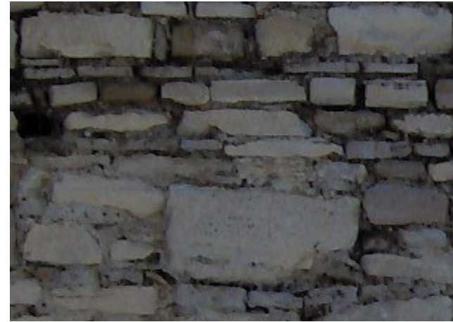
Figure 4.31. Progress of the efflorescences and discharge of mortar between the years 2004-2005
