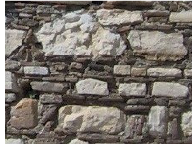
Figure 4.37. Progress of the black crust and discharge of mortar between the years 2003-2005
