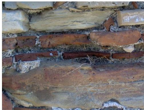
Figure 4.19. Discharge of mortar
