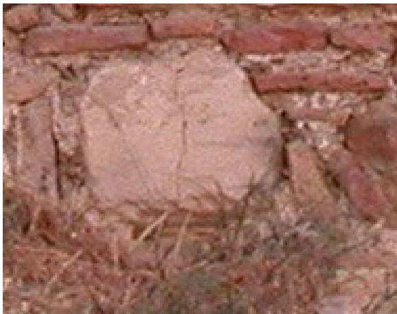
Figure 4.37. Progress of the black crust and discharge of mortar between the years 2003-2005
