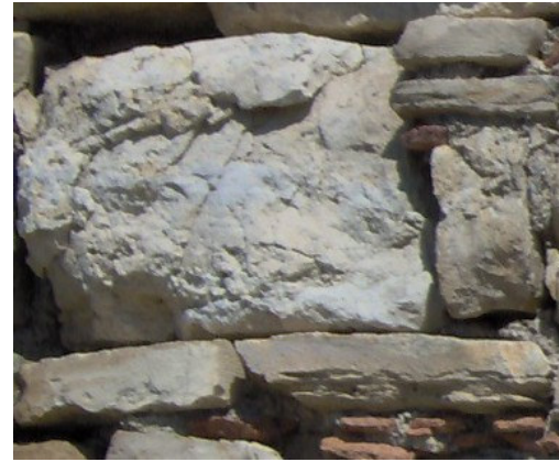
Figure 4.35. Progress of the splintering between the years 2003-2005
