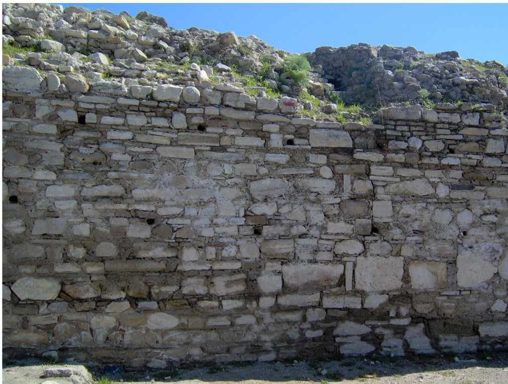
Figure 4.23. The state of deteriorations in recently excavated parts
