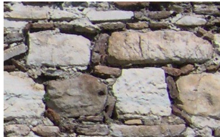
Figure 4.29. Progress of the black crust and discharge of mortar between the years 2002-2005
