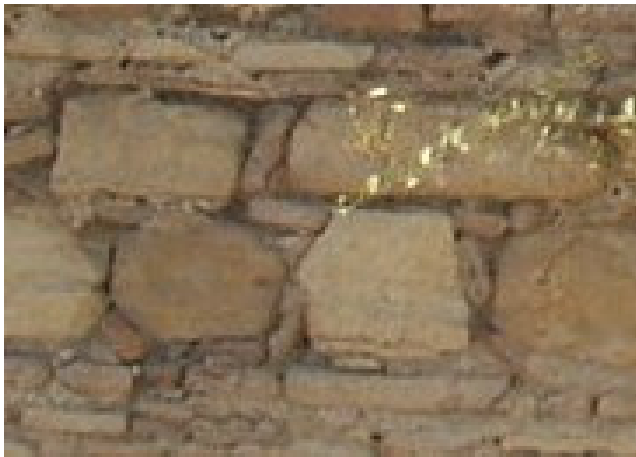
Figure 4.29. Progress of the black crust and discharge of mortar between the years 2002-2005
