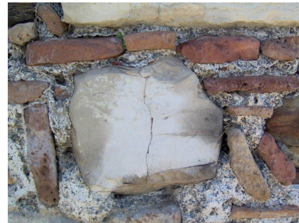
Figure 4.37. Progress of the black crust and discharge of mortar between the years 2003-2005
