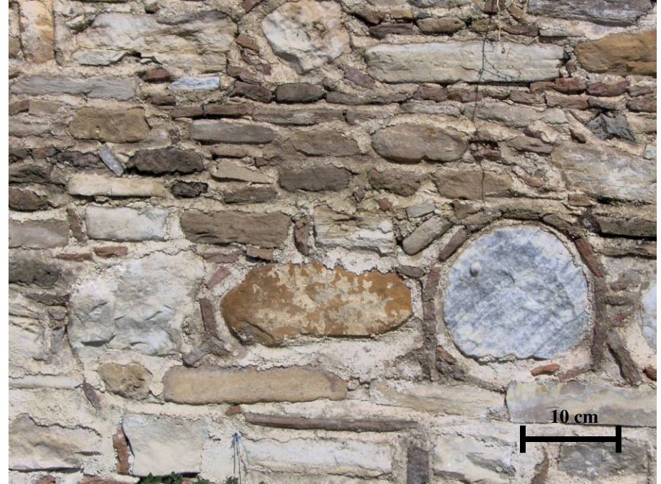
Figure 4.25. Progress of the colored and dark crust tracing the surface and discharge of mortar between the years 2003-2005
