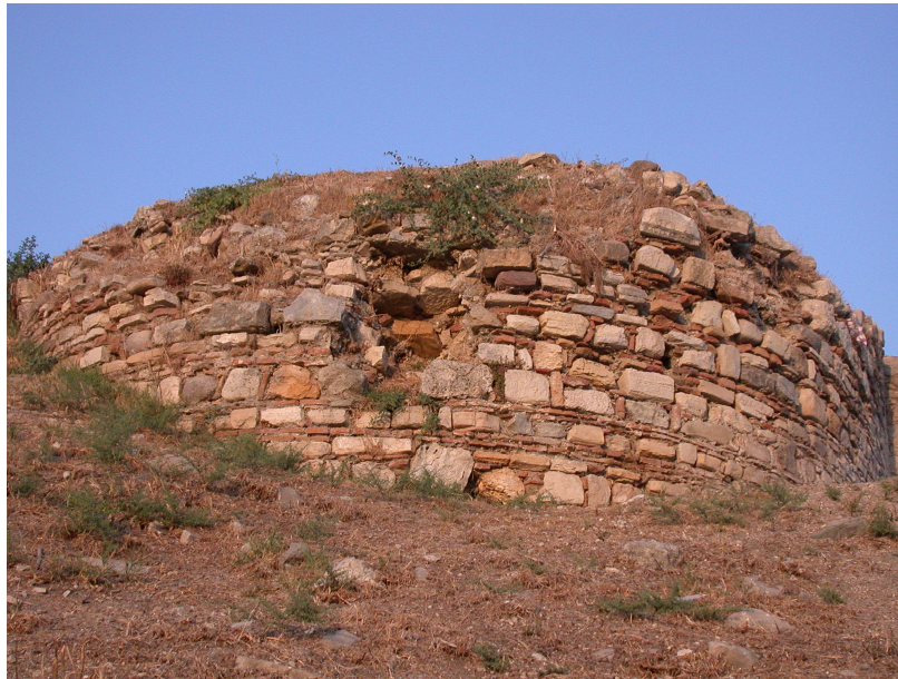
Figure 4.24. Discharge of mortar and break out
