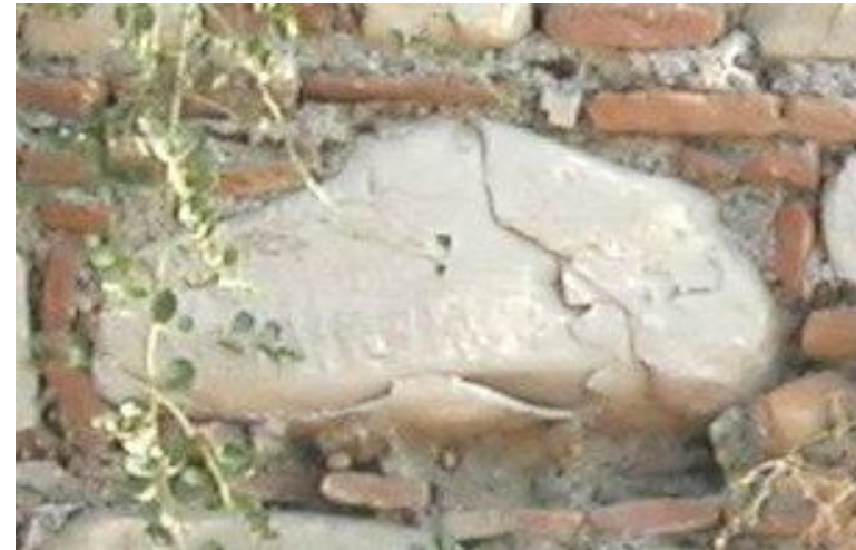
Figure 4.31. Progress of the efflorescences and discharge of mortar between the years 2004-2005
