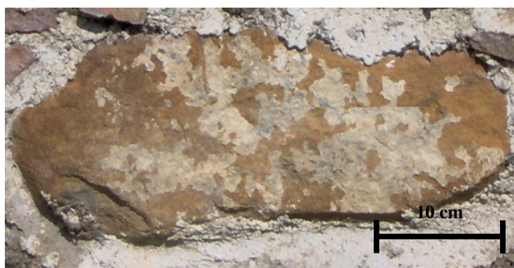
Figure 3.18. Colored crust tracing the surface
