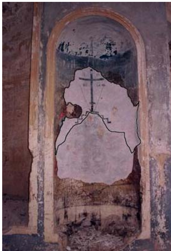
Figure 5.39. Loss of the paints due to the vandalism. Region bordered with red color was destroyed by human beings between 2003-2004 in order to discover the underlying cross figure
