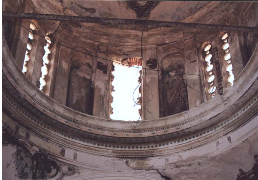
Figure 3.13. Wall paintings on the drum of the dome
