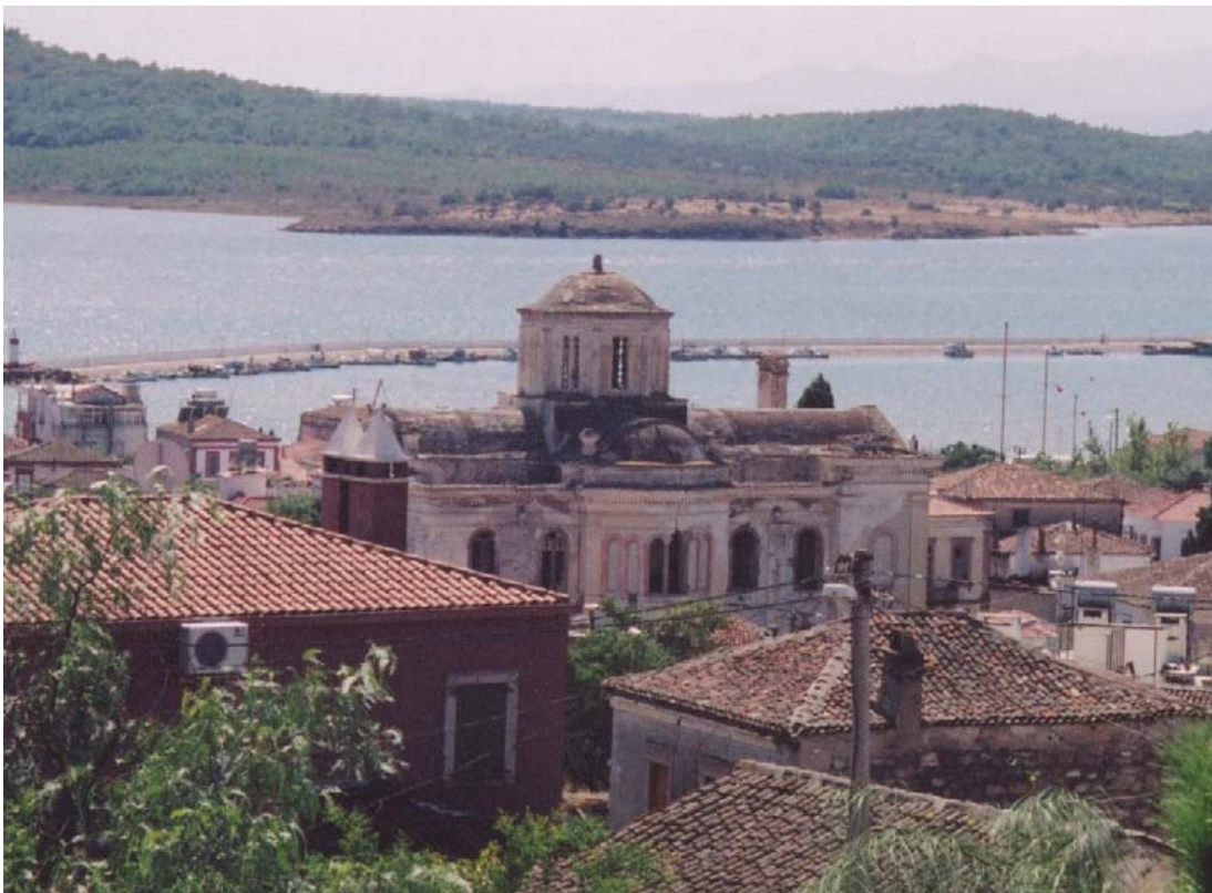
Figure 3.1. General view of the Taxiarhis Church
