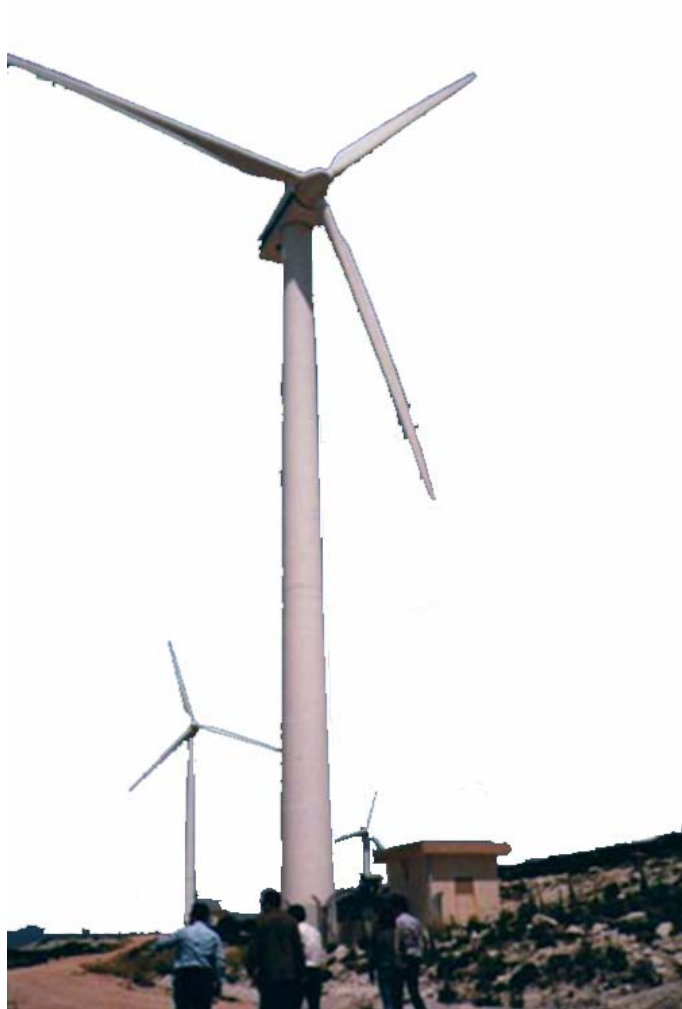
Figure 3.6. Horizontal axis wind turbines installed in Alacati/Turkey.
