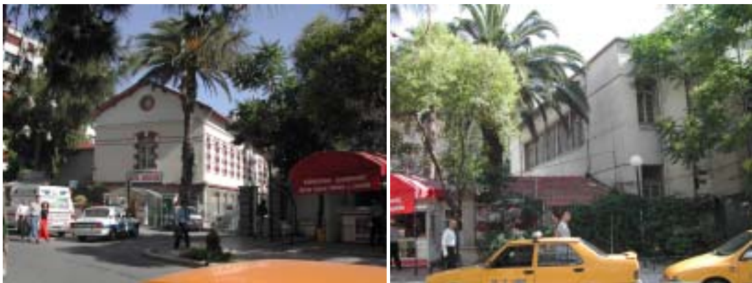
Figure 4.5 Street façade of hospital complex (the main building on the left, and the administration building on the right).
