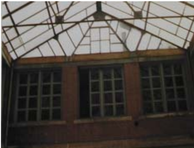
Figure 4.45 Shelter enclosing the courtyard top.
