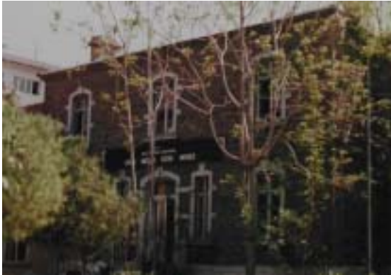
Figure 4.43 Building A entrance façade.
