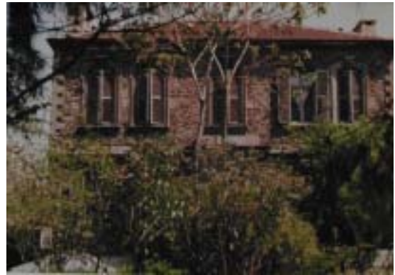
Figure 4.44 Building A side façade.
