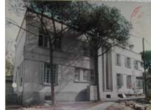
Figure 4.4 Side façade of the administration building.
