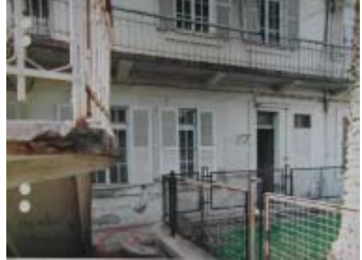
Figure 4.2 The old apartments demolished for the construction of new addition.
