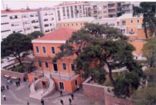
Figure 4.11 General view of Usakizade Mansion with new additions at rear.
