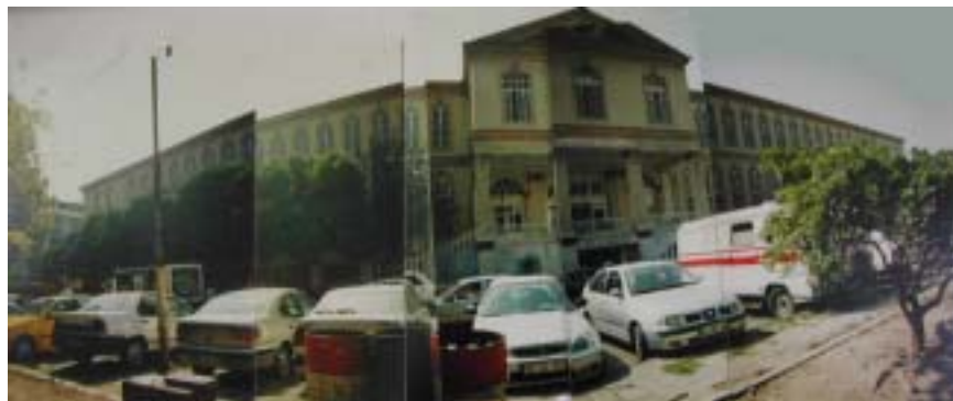
Figure 4.23 The entrance (north) façade of the hospital facing the Konak Square. (Source: Ministry of Culture and Tourism, Regional Directorate of Immovable Cultural And Natural Property in İzmir)
