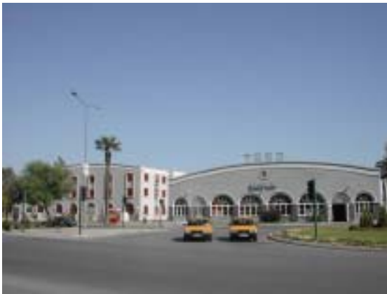
Figure 4.35 The Train Station with its new addition facing the main roads reaching Alsancak.
