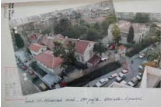
Figure 4.1 General view of Alsancak Public Hospital.
