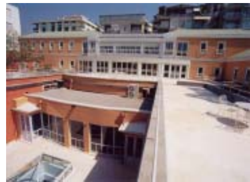
Figure 4.14 The courtyard façade of the new addition.
