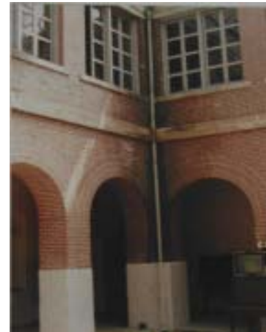
Figure 4.46 Arcade of the courtyard.
