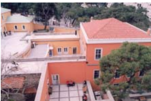
Figure 4.15 The connection of Usakizade Mansion with the new addition forming a small courtyard.
