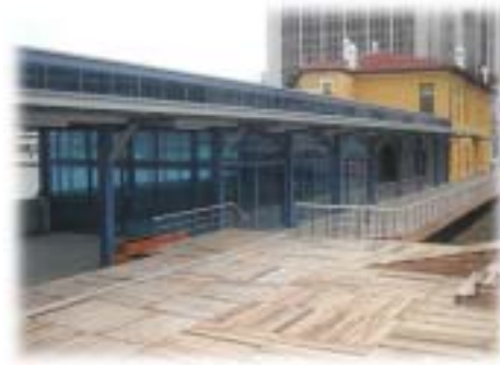
Figure 4.60 The new structure
