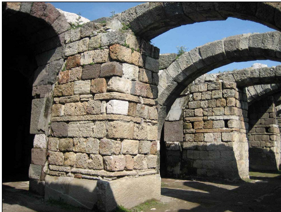
Figure 3.18. Abutments of arches which were strengthened subsequently.
