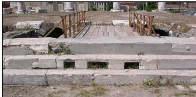
Figure 3. 21. Window openings through the steps of stylobate.
