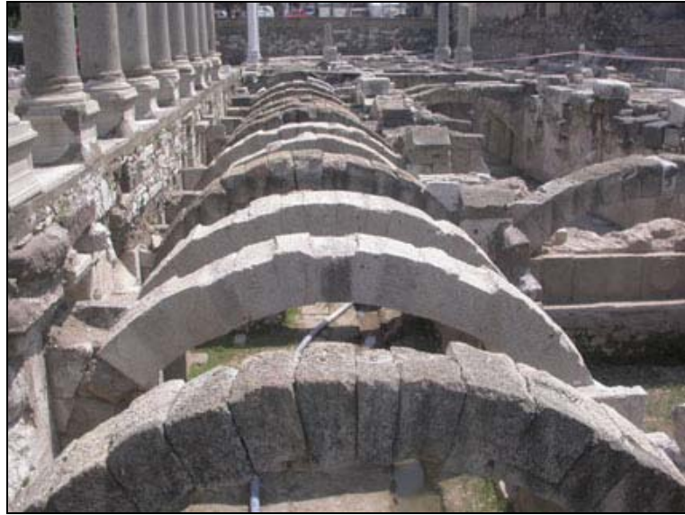
Figure 4.43. The state of the arches after the reconstruction implementation.
