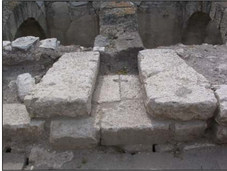
Figure 4.27. The 27th axis reveals the construction technique of the 5th and 4th courses.
