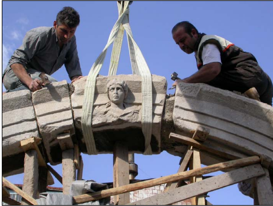
Figure 4.10. The disassembling process of the West Gate. (Source: Archives of the Agora excavations, 2004)
