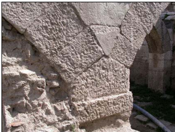
Figure 4.39. The west springer of the arches was for loading two arches.
