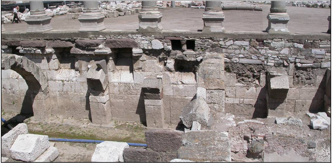
Figure 3.51. The east wall of the West Stoa completed with rubble and concrete.
