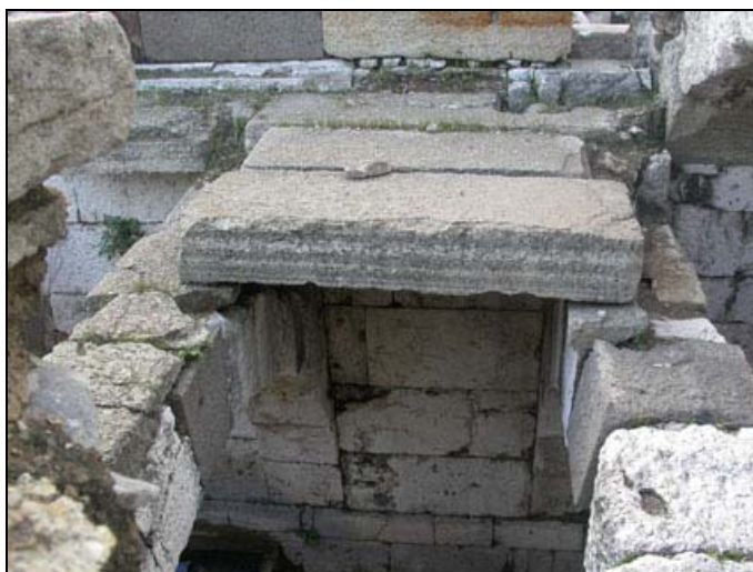
Figure 3.22. Flooring system bearing on the arches.
