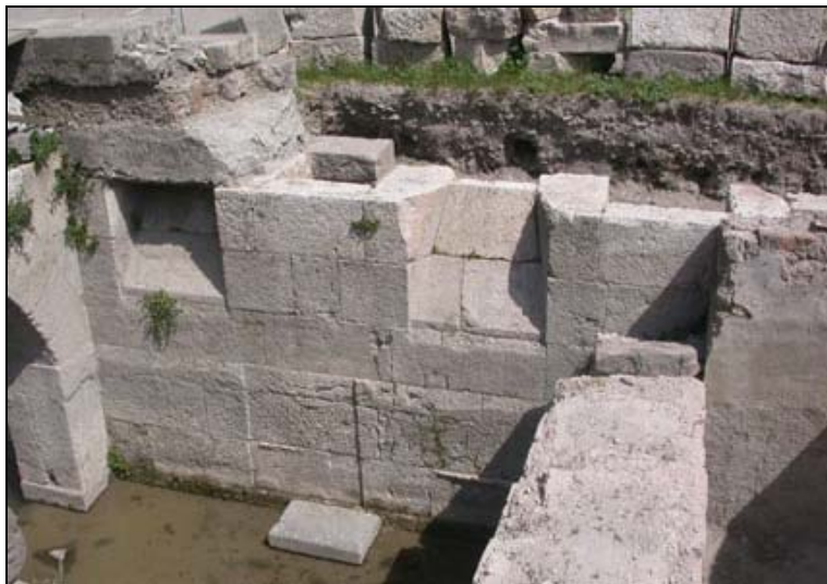
Figure 4.25. The east wall of the West Stoa, after the removal of the stylobate at 23rd axis.
