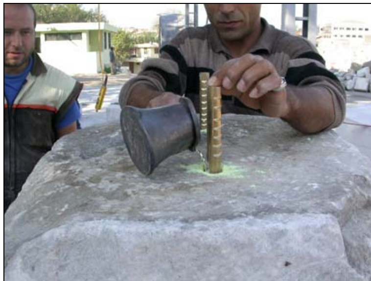
Figure 4.11. Bronze cylindrical clamps applied to the architectural pieces and surrounded with lead. (Source: Archives of the Agora excavations, 2004)
