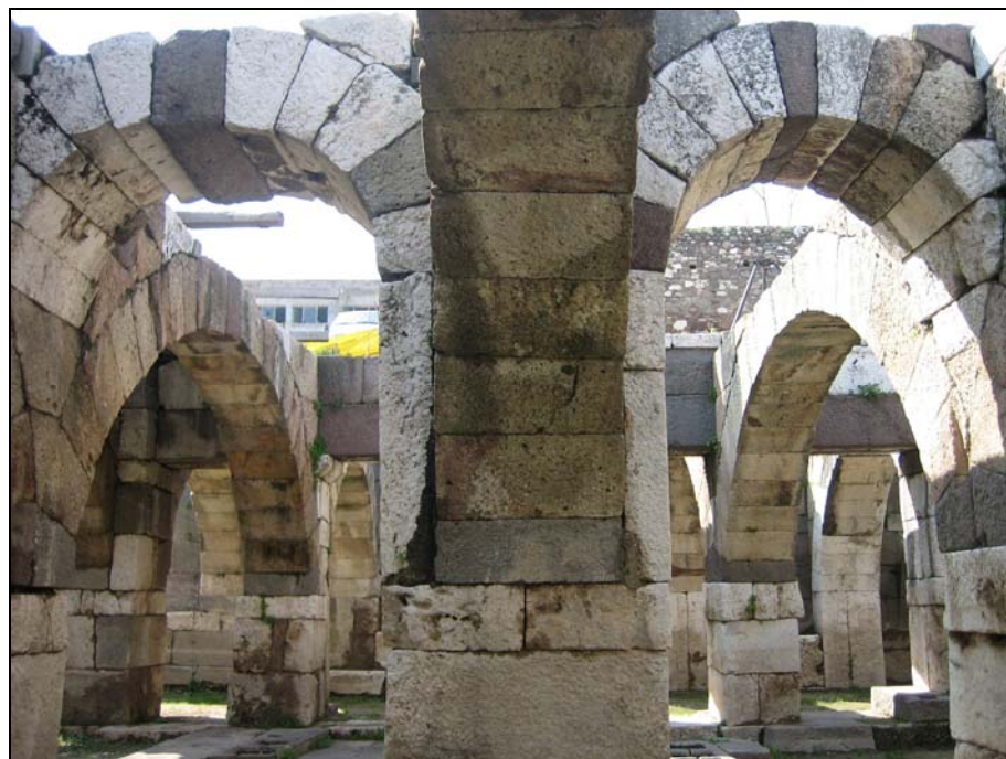
Figure 3.35. Each arch abutment is connected to the next with a smaller arch.
