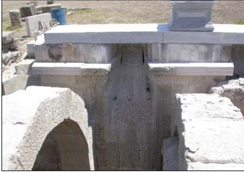
Figure 4.35. Reconstruction implementation of the window between 23 rd and 24 th axes.
