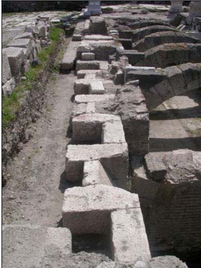
Figure 4.24. The construction style of the wall revealed after the removal of the concrete stylobate implementation.
