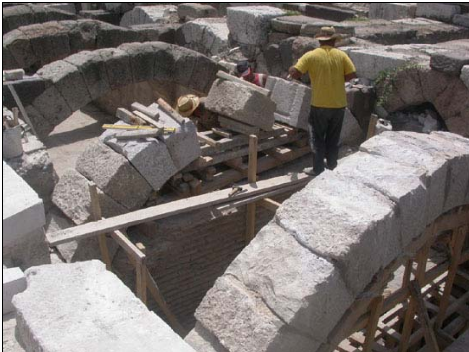
Figure 4.42. The reconstruction process of the arches. (Source: Archives of the Agora excavations, 2005)
