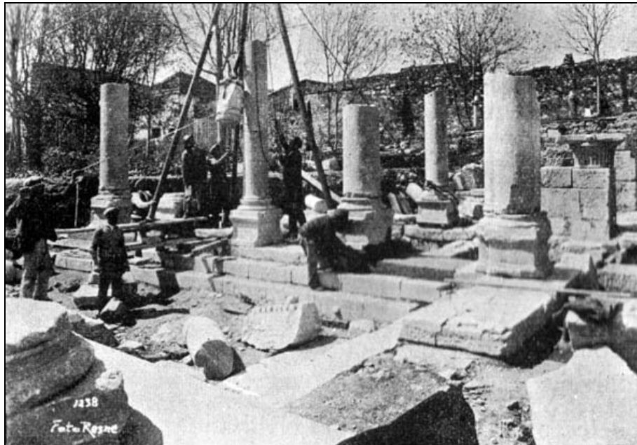
Figure 3.44. The completion of the missing parts by concrete. (Source: Archives of the Agora excavations)
