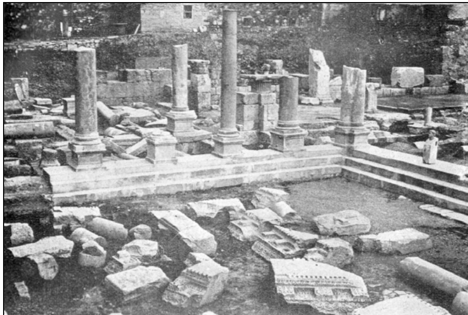
Figure 3.55. The missing parts were completed with concrete. (Source: İzmir Muhipleri Cemiyeti 1934)
