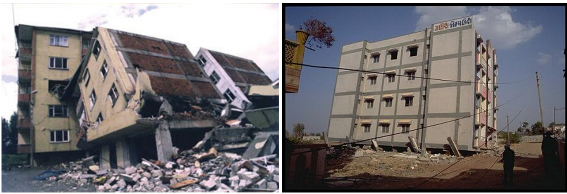
Figure 4.1. Soft Floor Effect
