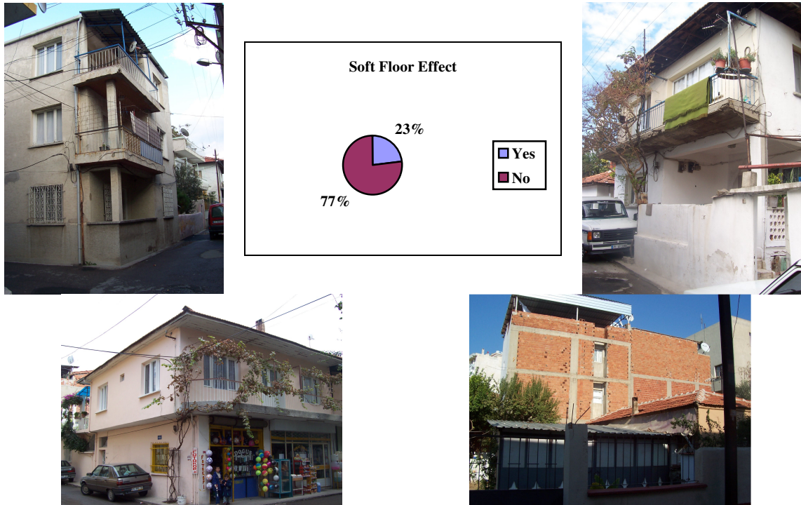
Figure 5.19. Soft Floor Effect
