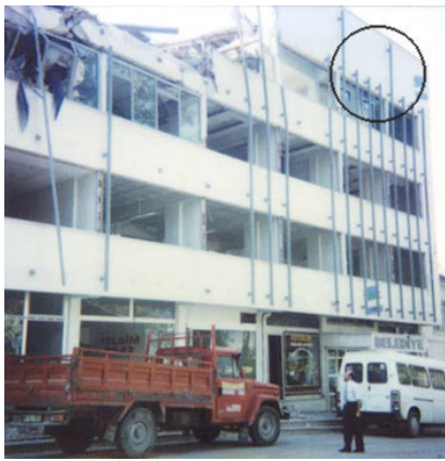
Figure 4.2. Short Column Effect
