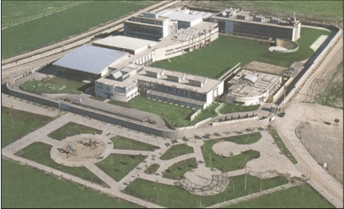
Figure 14. Aerial view of the Işıkkent ES campus (Karabey, 2004).
