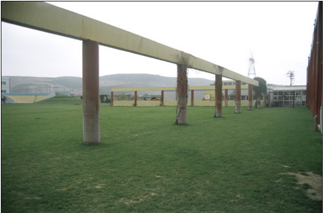
Figure 37. In the garden of Işıkkent ES, a row of columns provides a buffer zone in front of the windows of classrooms.
