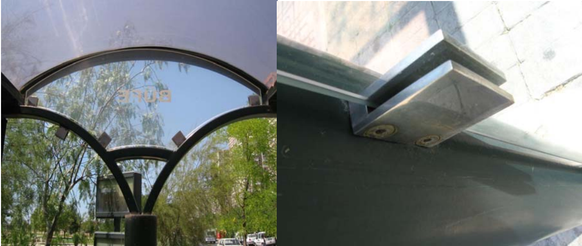
Figure 5.23. Junction detail
