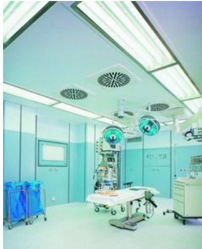
Figure 3.9. The use of PVC sheeting in operating room because of its hygienic property.
