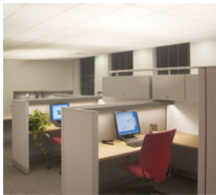
Figure 3.8. An Office with indirectly lighted ceiling.
