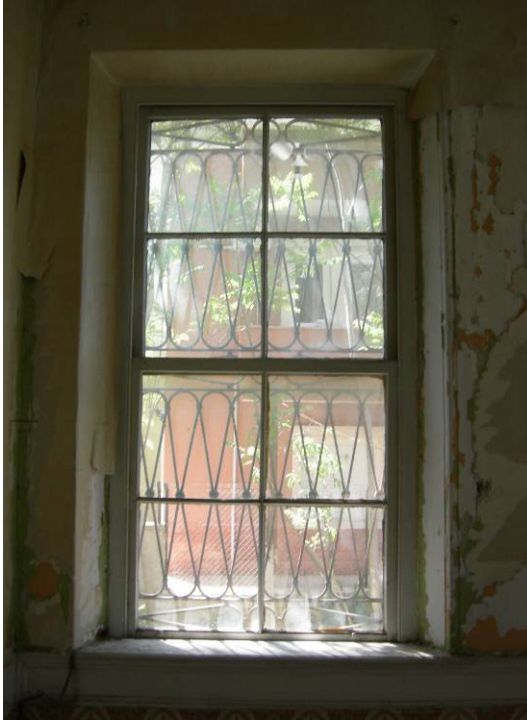
Figure 2.94. The room window viewed from the interior.
