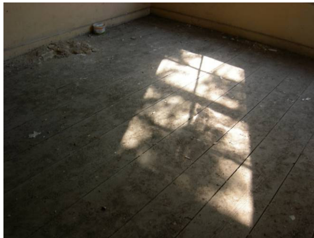
Figure 2.69. The timber floor covering of room 5 at the first floor.
