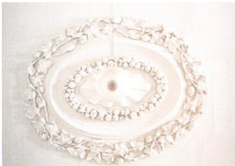
Figure 3.104. The gypsum ceiling ornaments at Latife Hanım House in Köprü. (Source: Kabaoğlu et al. 1999)
