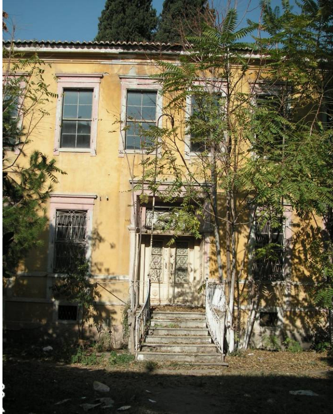
Figure 2.78. The southern facade of the house.
