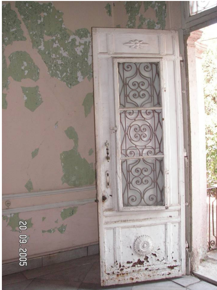
Figure 2.98. The leaf of the iron entrance door.
