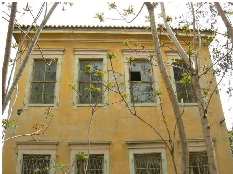
Figure 2.119. The distribution of openings on the western wall.
