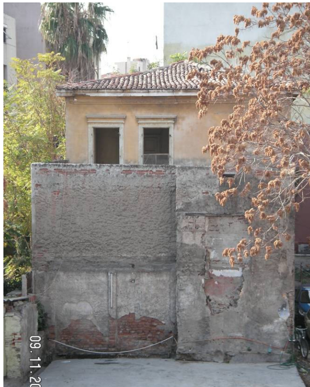
Figure 2.92. The eastern facade of the building.
