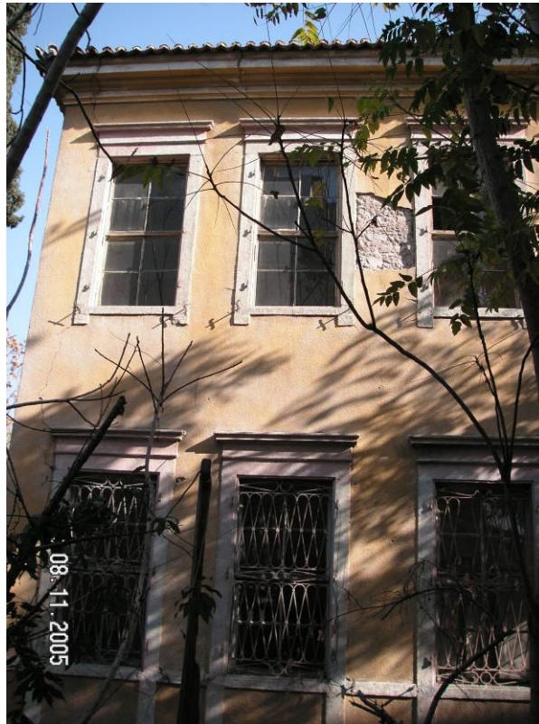
Figure 2.85. The western facade of the house.
