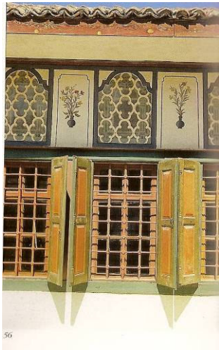
Figure 3.52. Upper and the lower level windows. (Source: Günay 1997)
