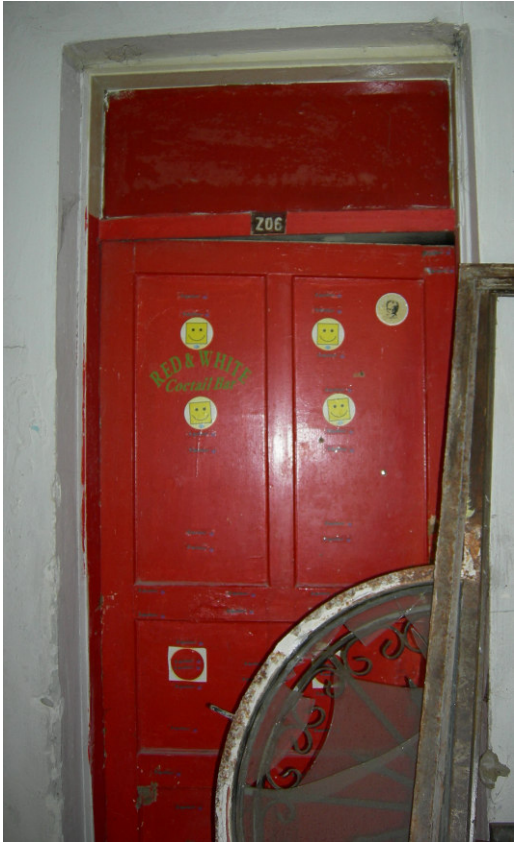
Figure 2.48. The door providing entrance to room 1 of the annex.
