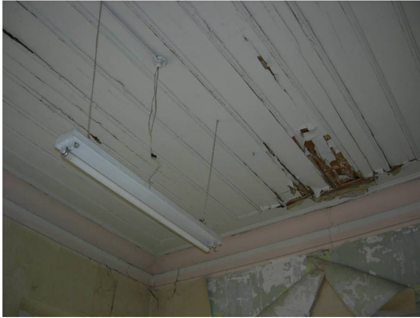
Figure 4.7. The ceiling of room1.
