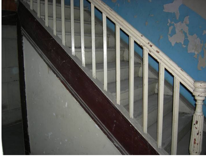
Figure 2.116. The renewed balusters.
