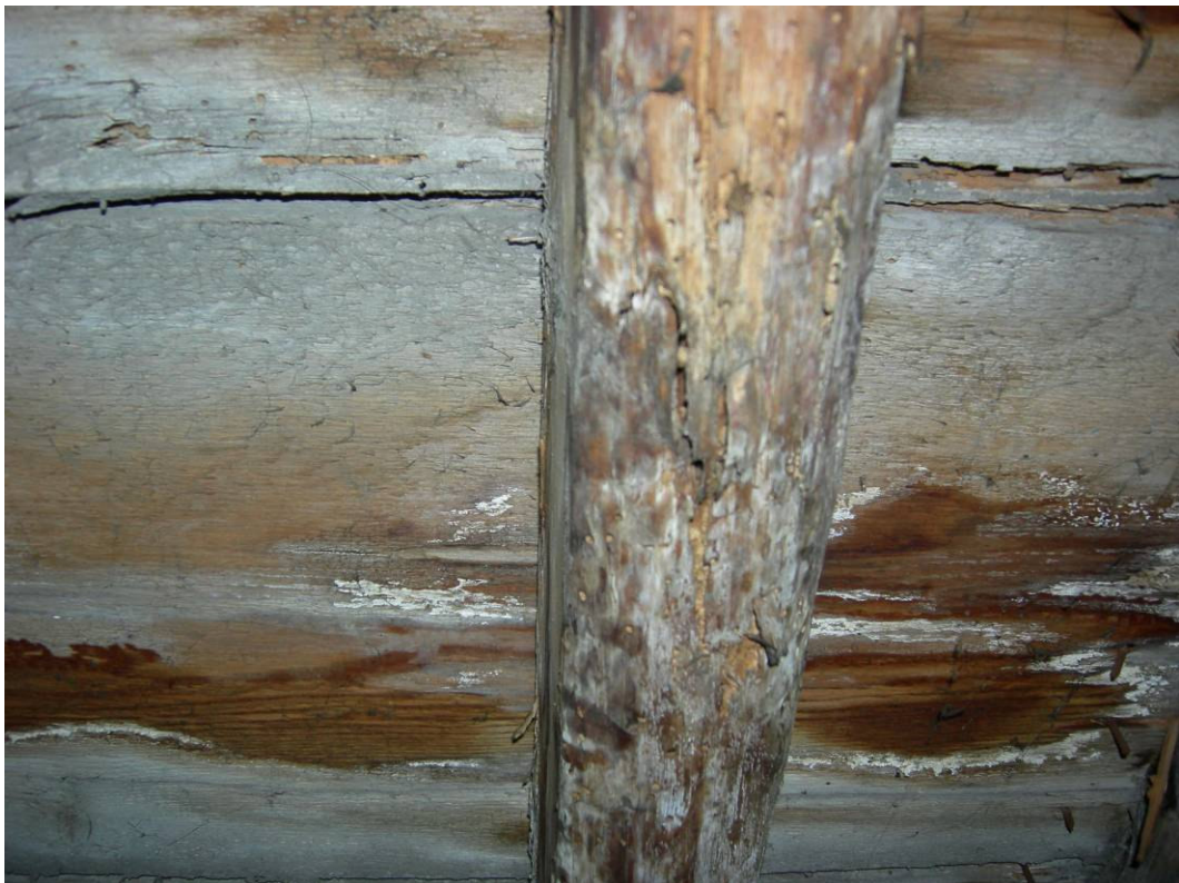
Figure 2.125. Holes in the timber beam, white stains in the timber covering at the basement.
