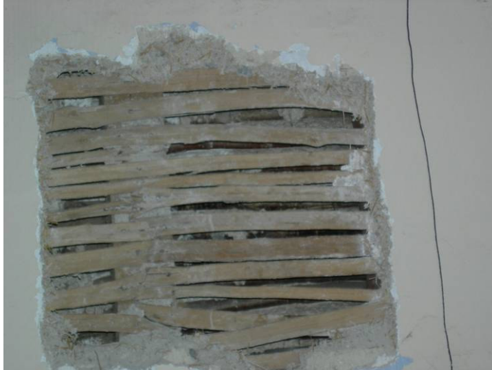
Figure 2.120. The northern wall of room 6.
