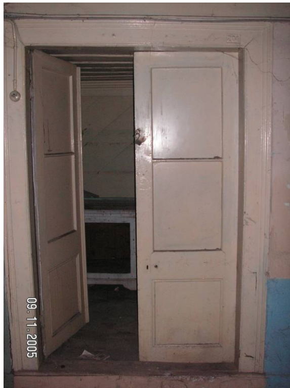
Figure 2.40. The door between the kitchenette and the stairwell.
