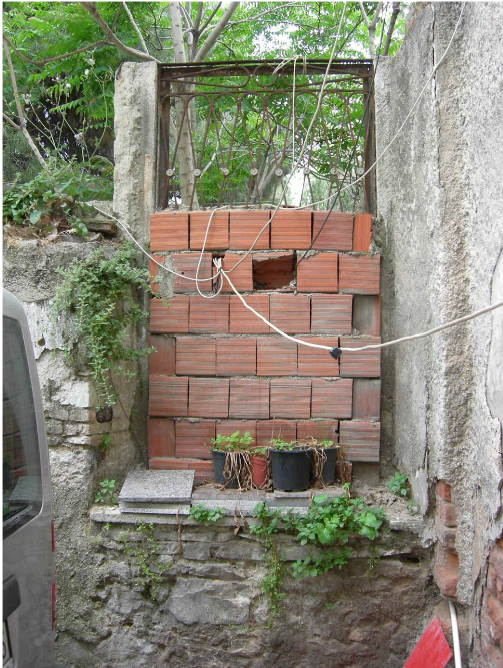
Figure 2.111. The masonry wall piece at the south of the annex.
