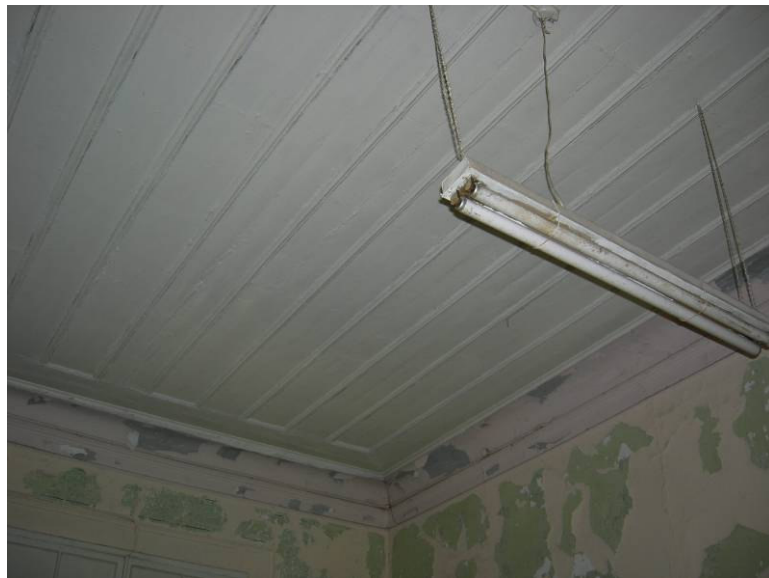
Figure 2.24. The ceiling of the inner hall covered with wood laths.
