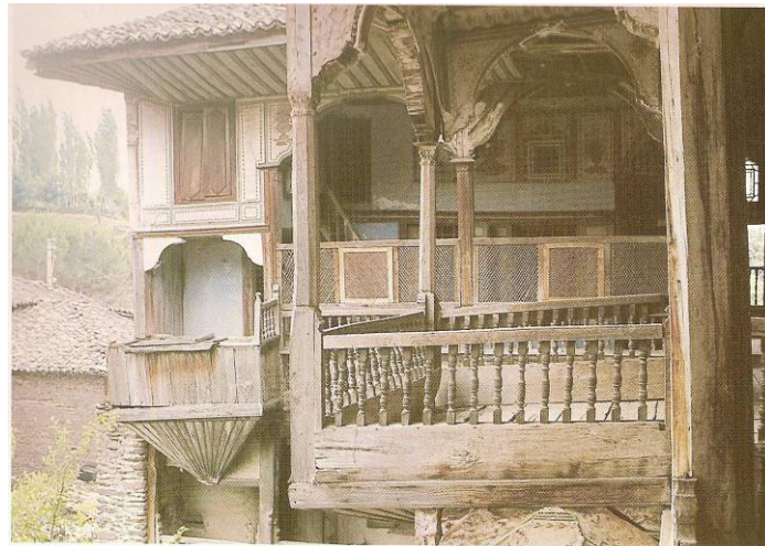
Figure 3.32. Projections from the open hall of Çakırağa Mansion. (Source: Kuban 1995)
