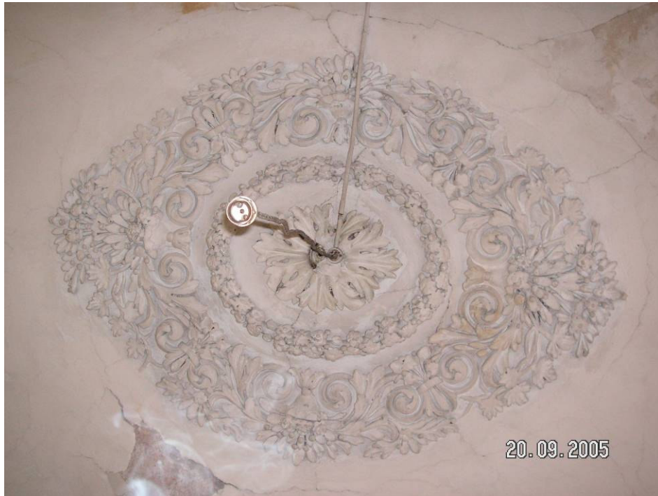
Figure 2.60. The stucco work in the center of the ceiling of the hall at the first floor.
