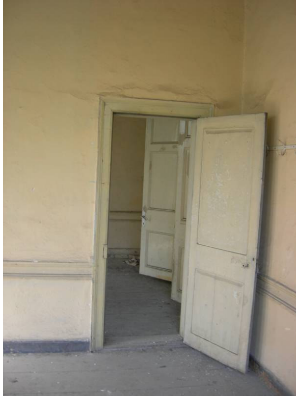
Figure 2.66. The door between the room 4 and room 5 at the first floor.
