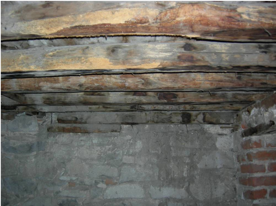
Figure 2.13. The ceiling of storage space 2 at the basement.
