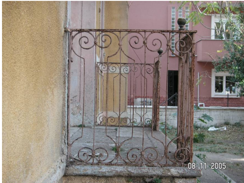
Figure 2.88. The iron guard rail of the northern terrace.
