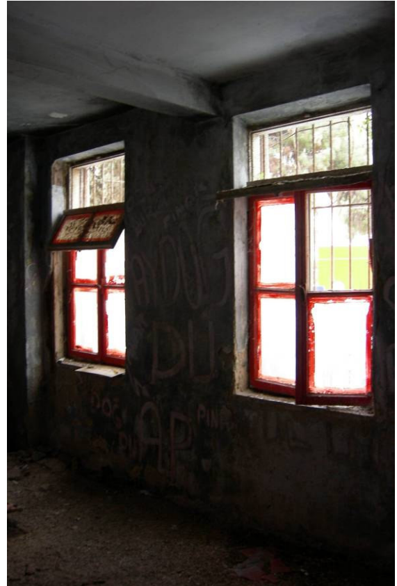
Figure 2.49. The windows on the northern wall of the annex.
