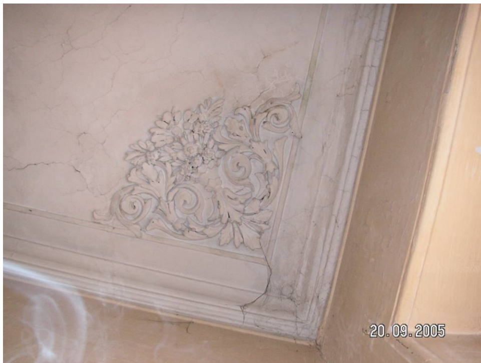
Figure 2.61. The molding and the stucco work at the corner of the ceiling of the hall at the first floor.
