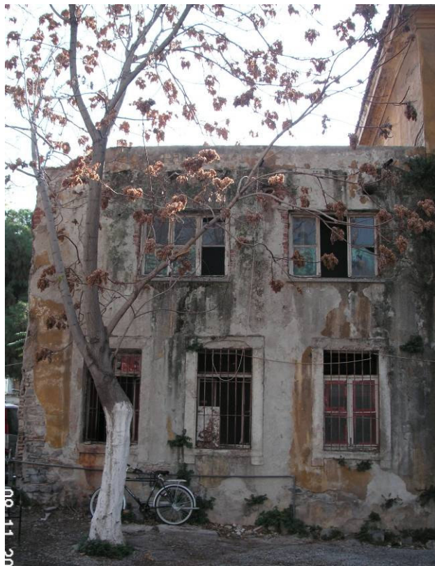
Figure 2.91. The northern facade of the annex.
