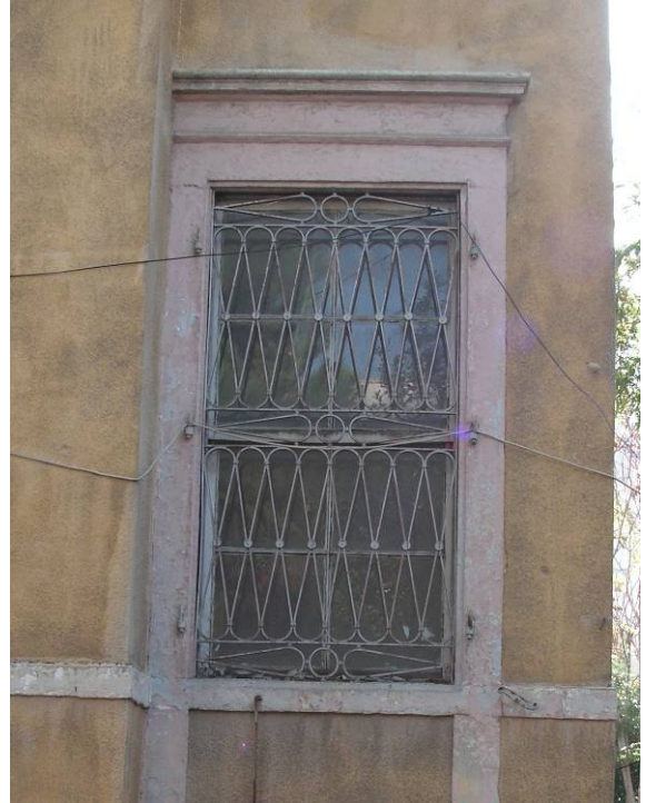
Figure 2.95. The room window viewed from the exterior.
