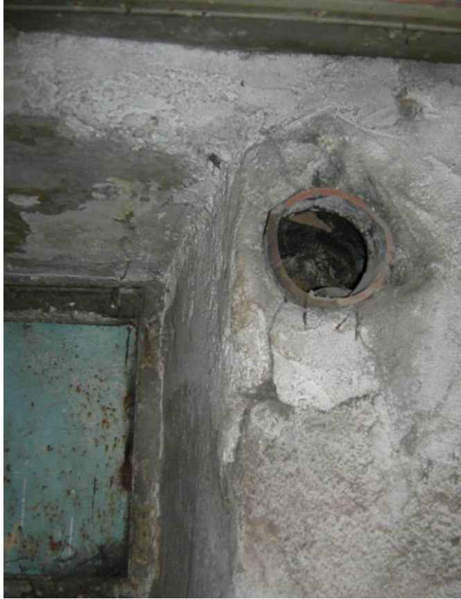
Figure 4.3. Ceramic pipe at the northern wall of the basement.
