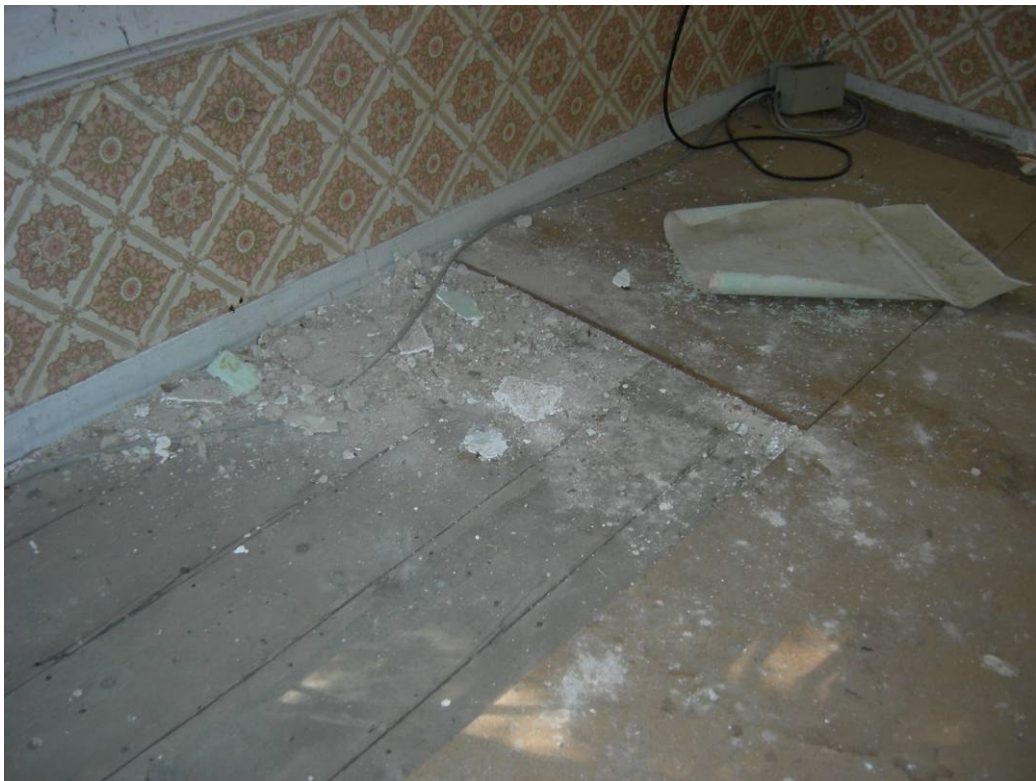
Figure 2.34. The floor covering of room 1.
