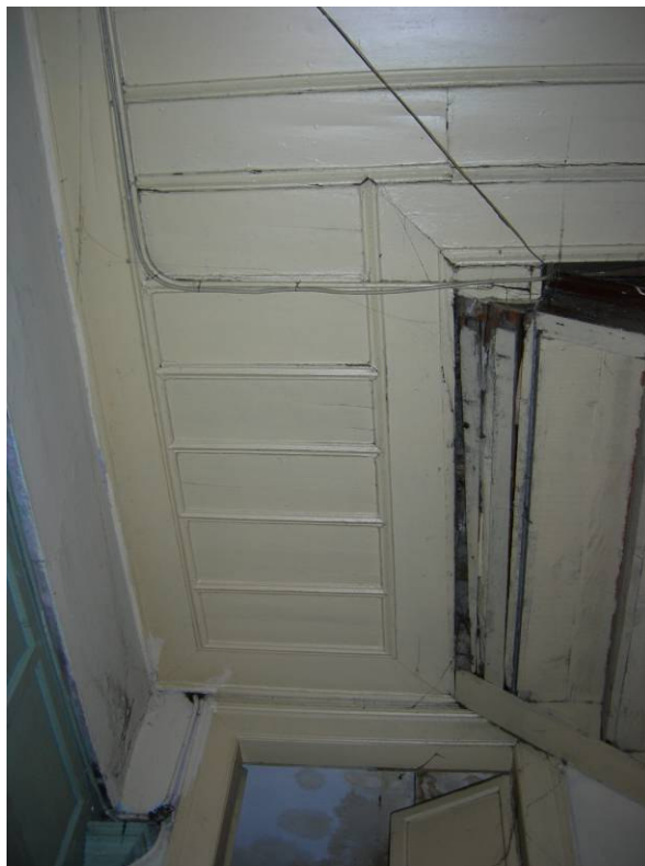
Figure 2.38. The ceiling covering of the stairwell.
