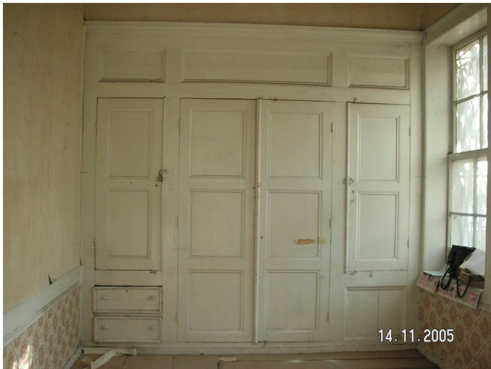
Figure 2.47. The cupboard in room 3.
