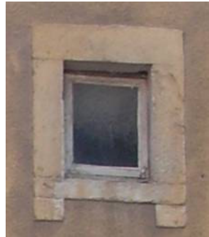
Figure 2.97. The window of the wet space viewed from the exterior.
