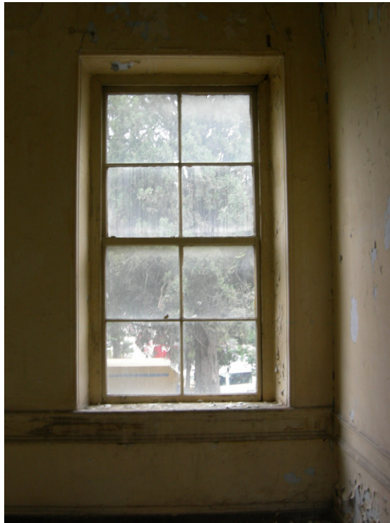
Figure 2.62. The window of the hall at the first floor.
