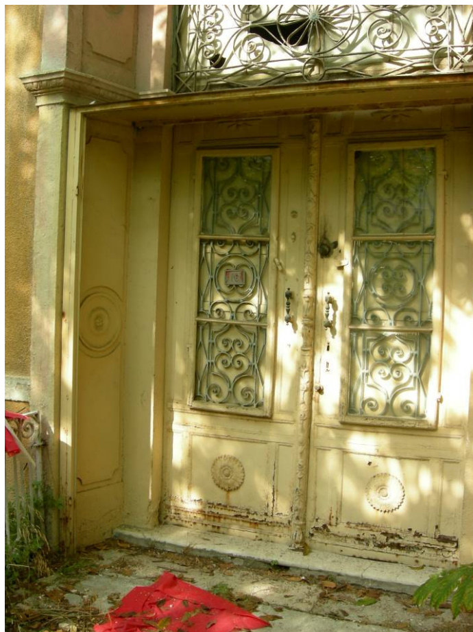
Figure 2.113. The additional metal joinery at the southern entrance.
