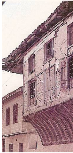
Figure 3.79. Timber skeleton with adobe infill. (Source: Bektaş 1996)
