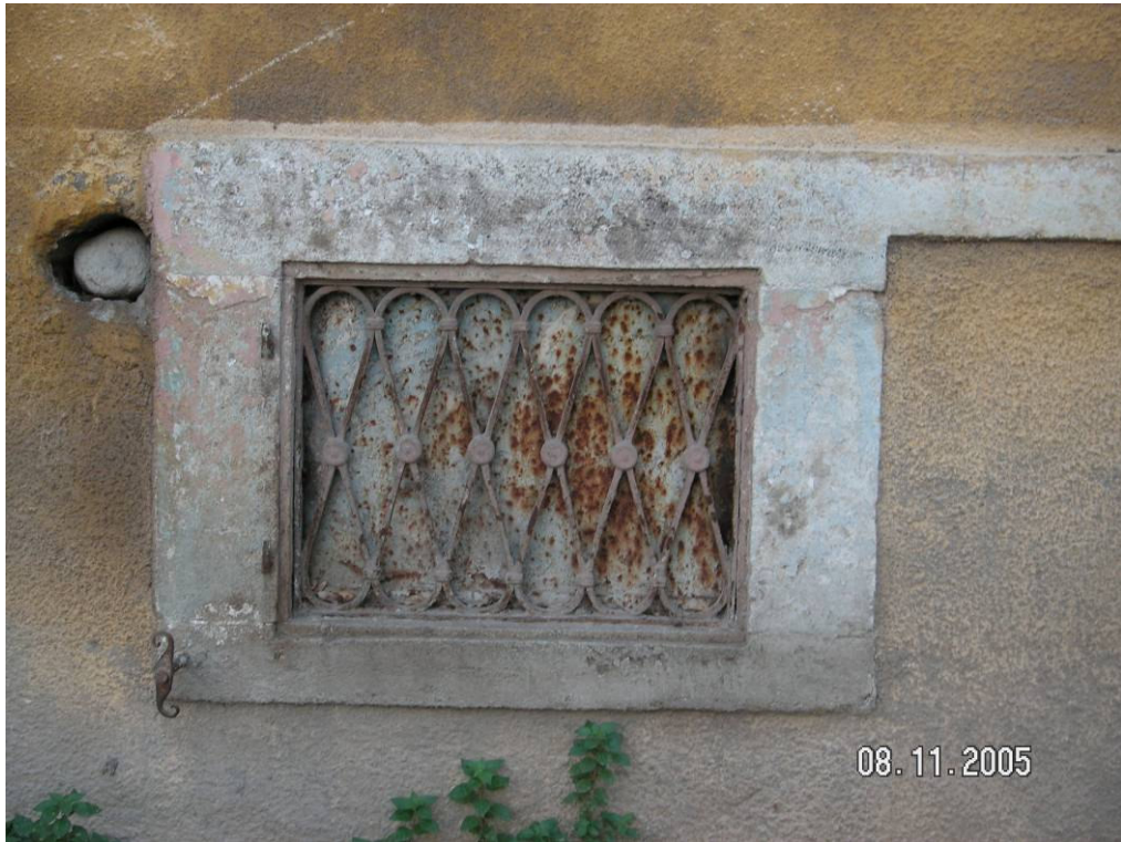
Figure 2.90. The rectangular shaped basement window.
