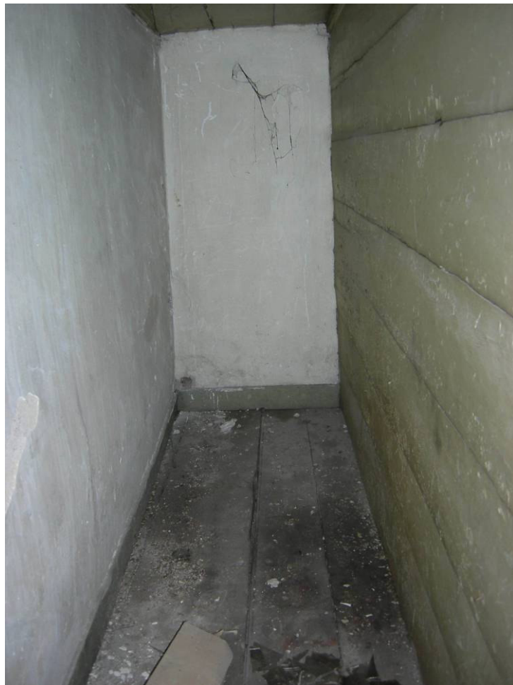
Figure 2.57. The dark space at the mezzanine floor.
