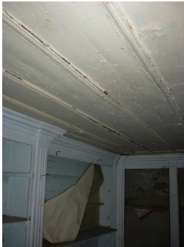
Figure 2.43. The kitchenette and its ceiling.
