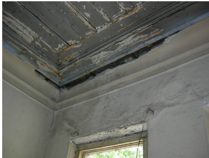
Figure 2.75. The ceiling of room 6 at the first floor.
