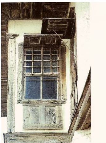
Figure 3.55. Shutters opening horizontally. (Source: Günay 1997)
