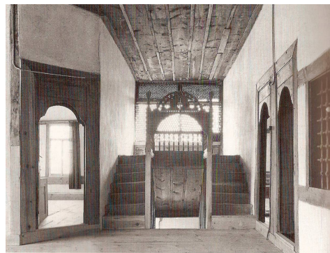
Figure 3.38. Stairs placed in the side hall. (Source: Günay 1997)
