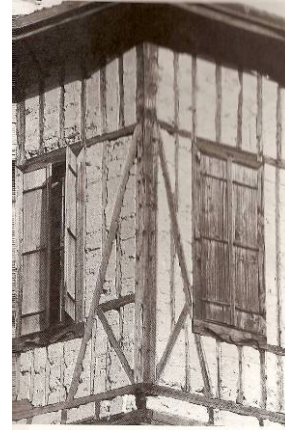
Figure 3.78. Timber skeleton with brick infill. (Source: Bektaş 1996).
