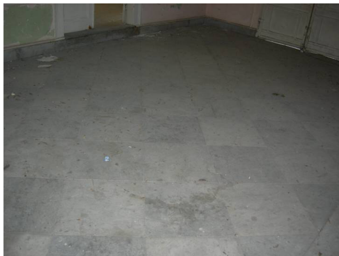
Figure 2.30. The floor covering of the inner hall at the ground level.
