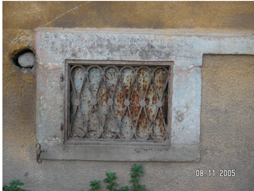
Figure 4.5. Shutter backstops of the windows of wet space 1 and 2 at the basement.
