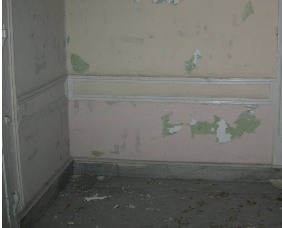
Figure 2.25. The timber chair rail running along the walls of the hall.
