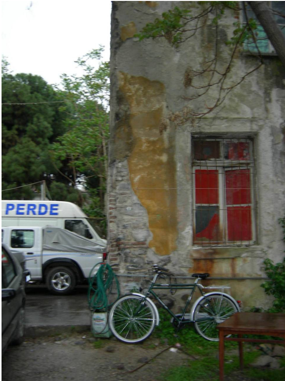
Figure 2.105. The north wall of the annex at the ground floor level.
