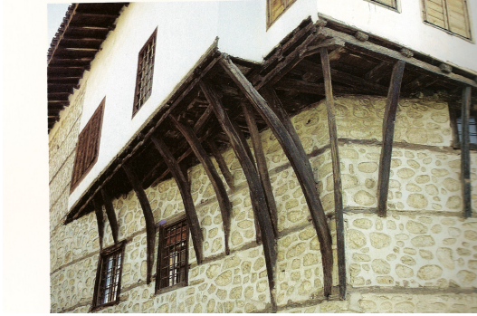
Figure 3.77. The horizontal lintels. (Source: Günay 1997)
