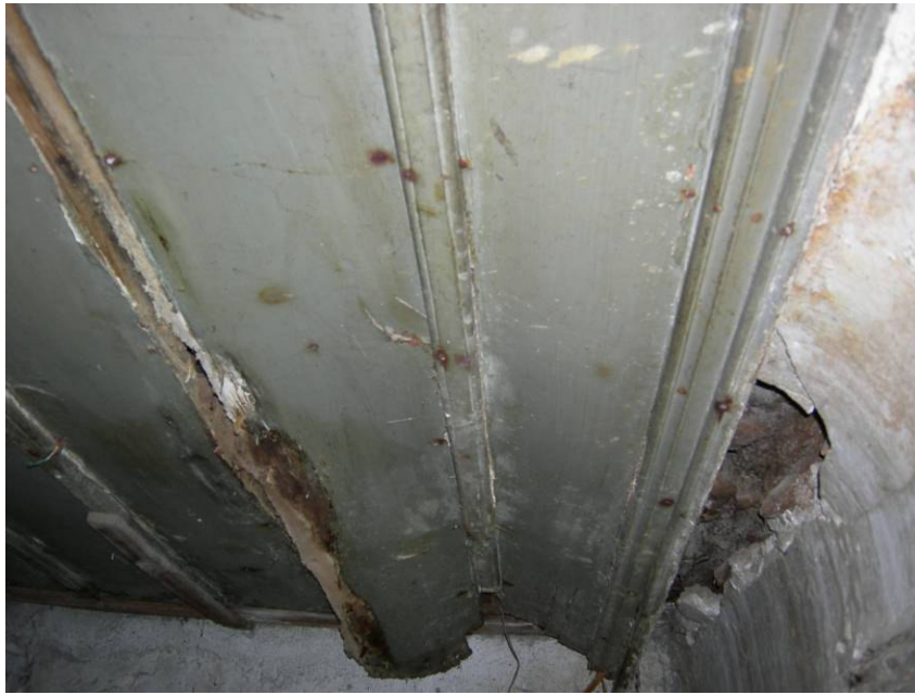
Figure 2.17. The ceiling of wet space 2 at the basement floor.
