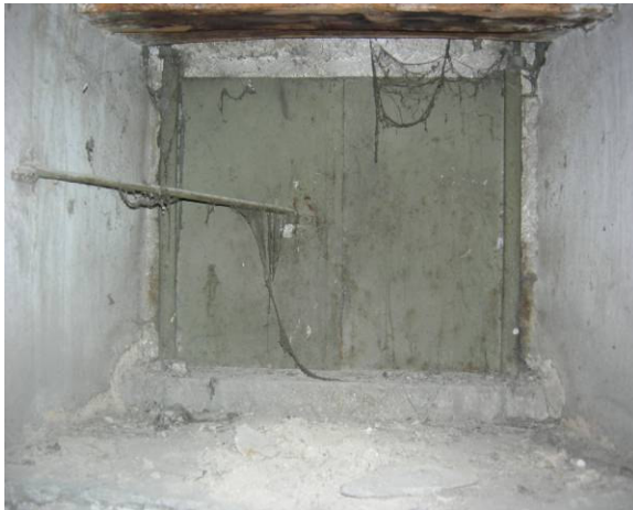
Figure 2.96. The basement windows viewed from the interior.
