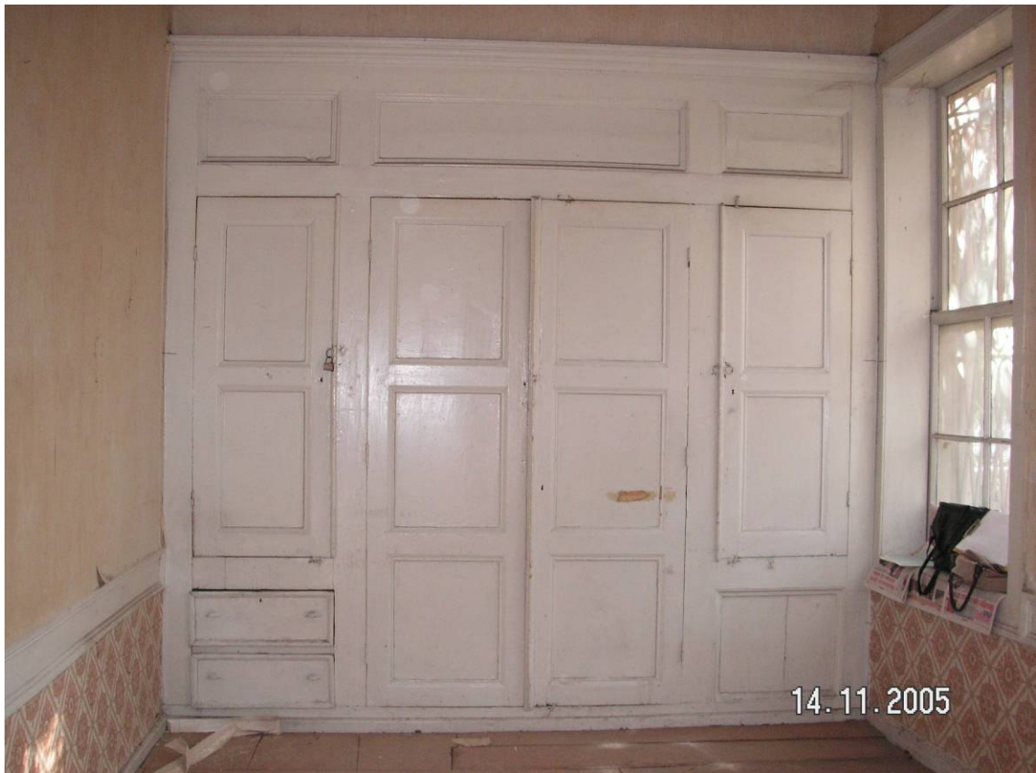
Figure 4.10. The cupboard in room 3.
