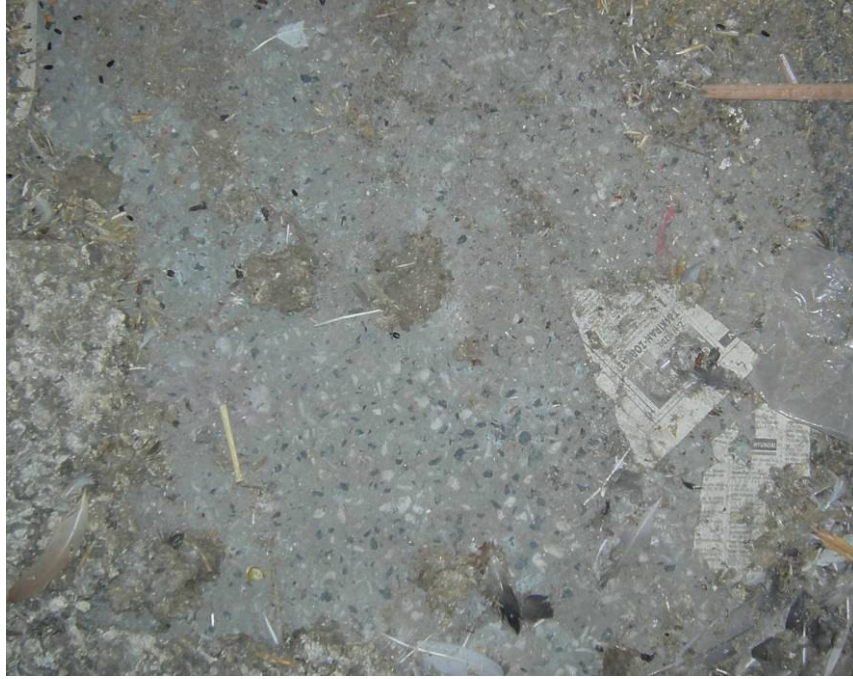
Figure 2.110. The floor of the annex covered with cast in place terrazzo at the ground level.
