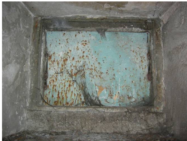
Figure 2.15. The window of wet space 1 at the basement floor.
