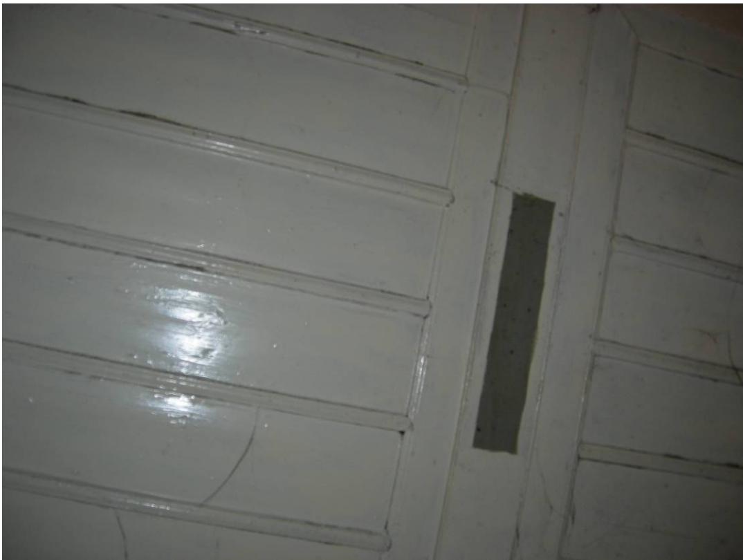
Figure 2.73. The ceiling of the wet space at the first floor.
