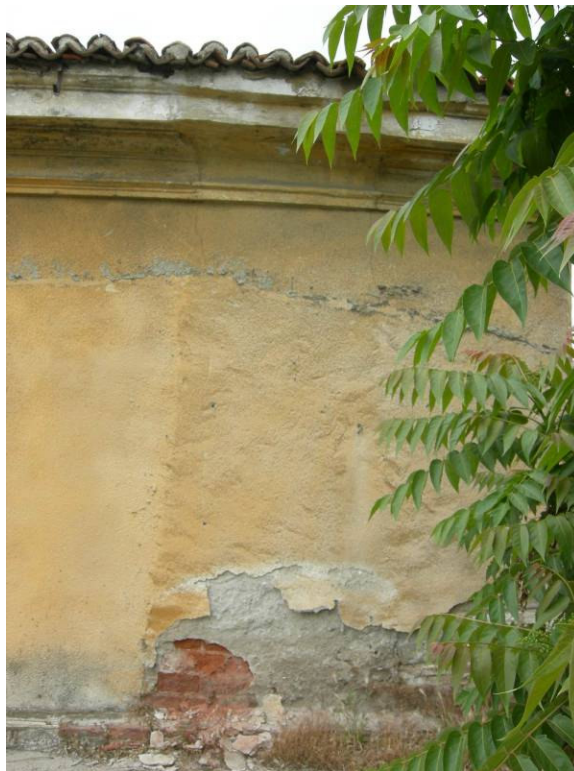
Figure 4.4. The trace of a fireplace on the east wall of the house.
