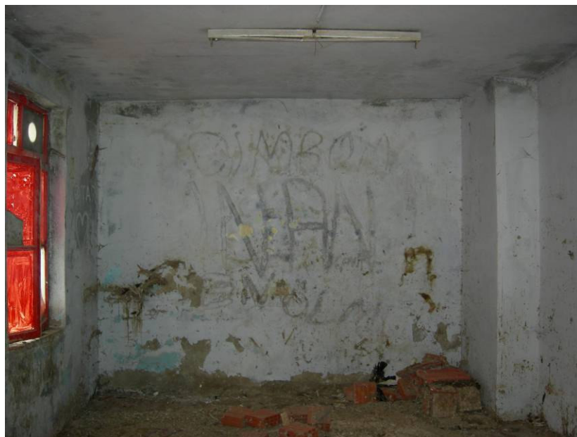
Figure 2.50. The walls and the ceiling of room 1 at the annex.
