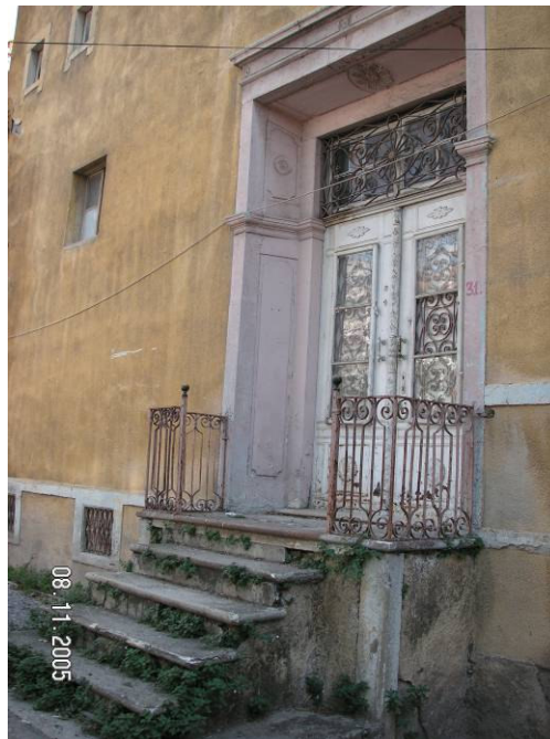
Figure 2.87. The elevated terrace and the recessed door at the north.
