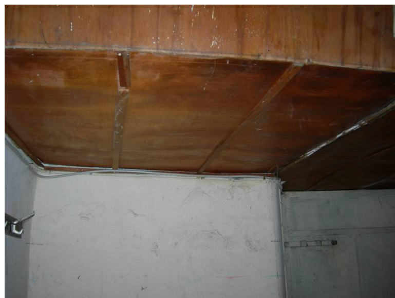
Figure 2.115. The renewed ceiling covering of space under the stair landing.
