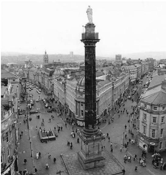
Figure 3.47. GMA before Refurbishment (Source: Akkar 2005b)
