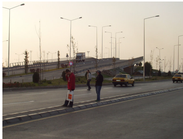
Figure 4.117. Viaduct at the south part of the Square, 21.11.06
