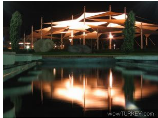
Figure 74. View from pedestrian platform (Source: WEB_36 2006)
