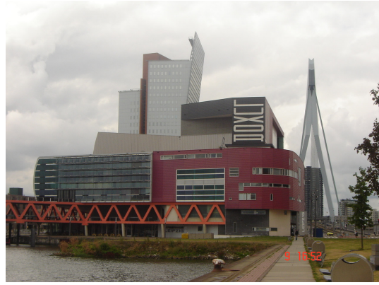
Figure 42. View of Luxor Theater (Source: Personal archive)
