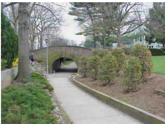
Figure 6. The pedestrian tunnel seen from B-Park (Source: WEB_10 2006)
