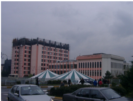
Figure 82. View from municipality building (Source: Personal archive)
