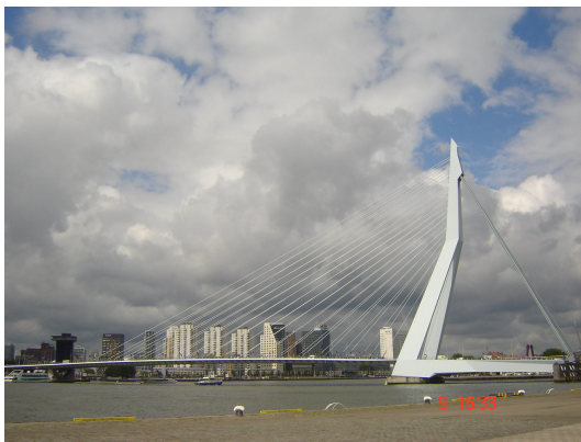
Figure 37. View of Erasmus Bridge (Source: Personal archive)
