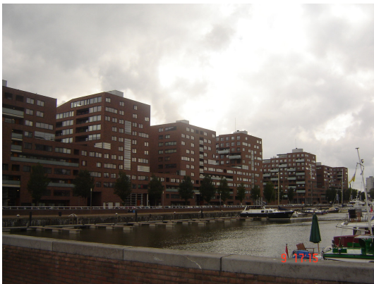
Figure 45. View of housing blocks in Landtong (Source: Personal archive)
