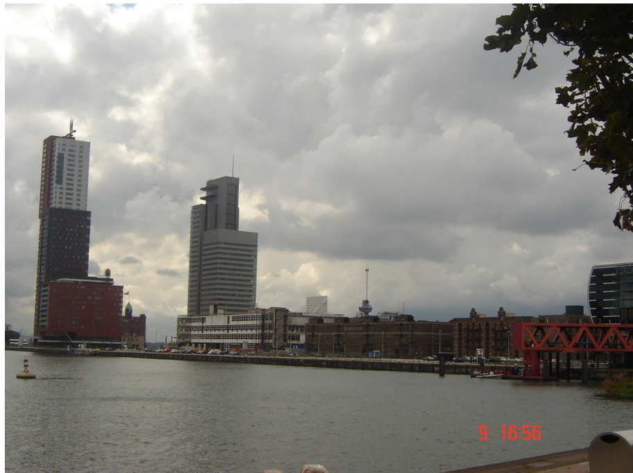
Figure 16. View of Wilhelmina Pier (Source: Personal Archive)
