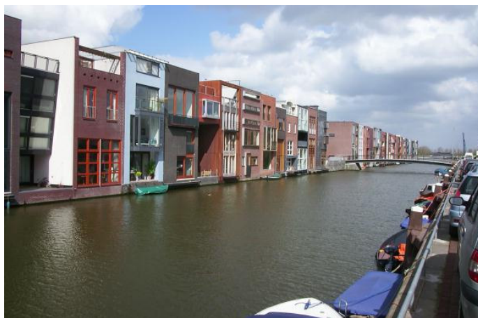
Figure 23. View from housing units from inner canal (Source: WEB_27 2006)
