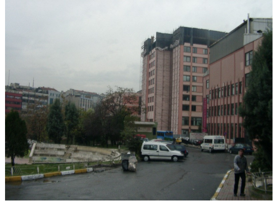
Figure 85. View from the service area (Source: Personal archive)
