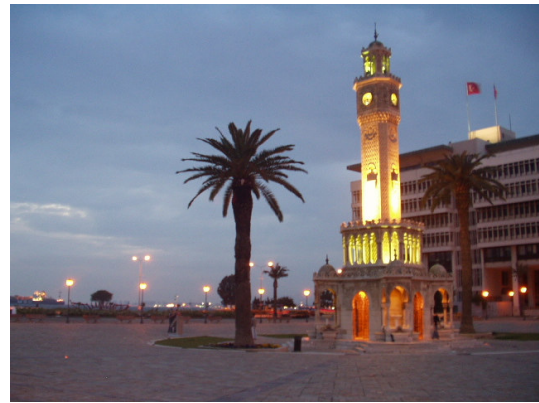
Figure 68. View of historical tower at night (Source: Personal archive)
