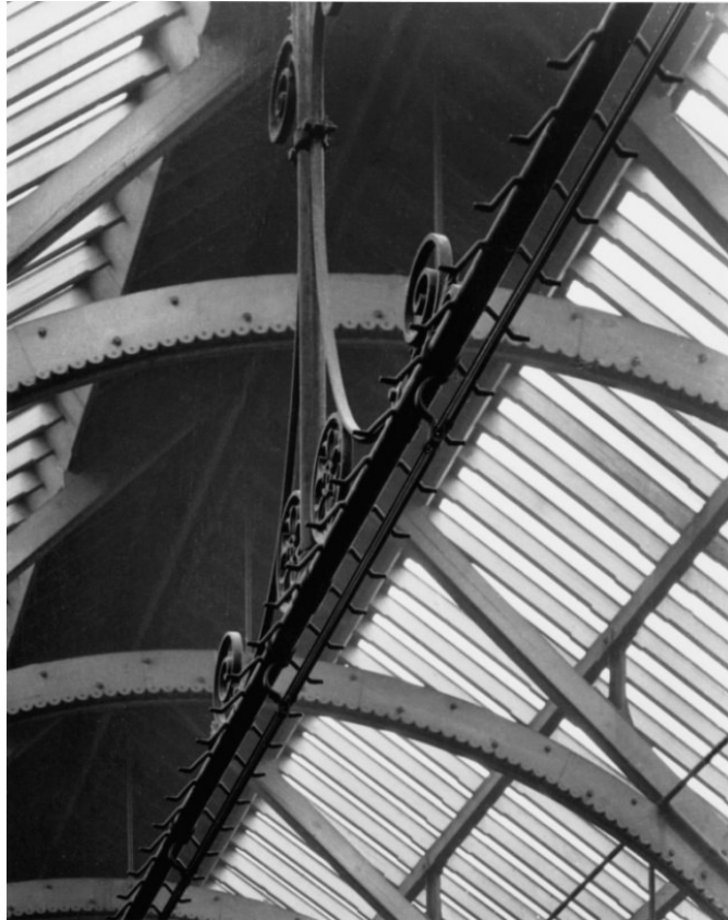
Figure 4.1. Detail of a gas pipe, showing the burners on both sides. (Source: Swinney 1999)
