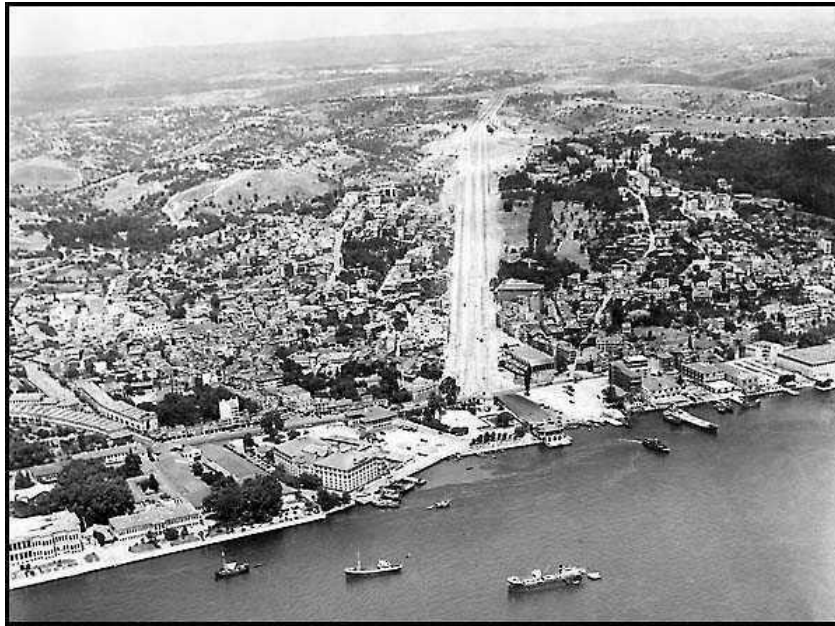
Figure 4.7. Construction of Barbaros Boulevard from Beşiktaş (Source: WEB_10)
