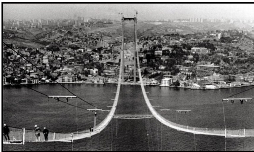
Figure 4.6. Bosphorus Bridge in Construction
