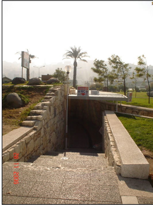
Figure 4.89. Entrance of public toilets
