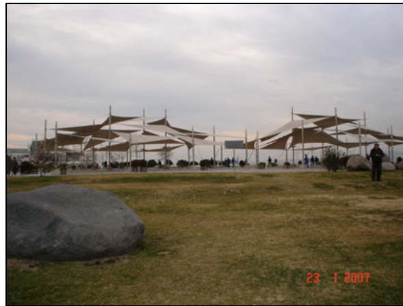
Figure 4.76. General view from sheltered area
