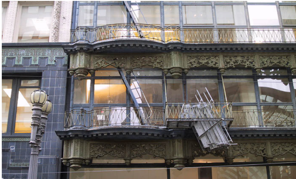
Figure 2.6. Facade Detail of Hallidie Building (Source: Brock 2005)
