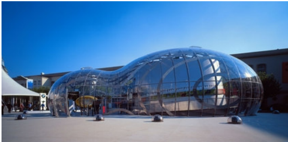
Figure 3.6. Franken, BMW pavilion (Source: Kolarevic 2005)
