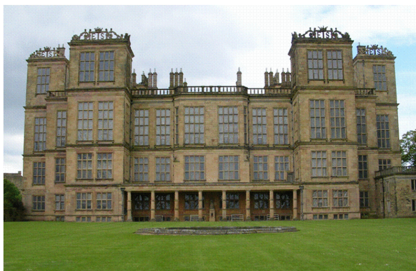
Figure 2.3. Bess of Harwick Mansion, large window openings from ceiling to floor occupies the function of cladding wall (Source: Quirouette 1982).
