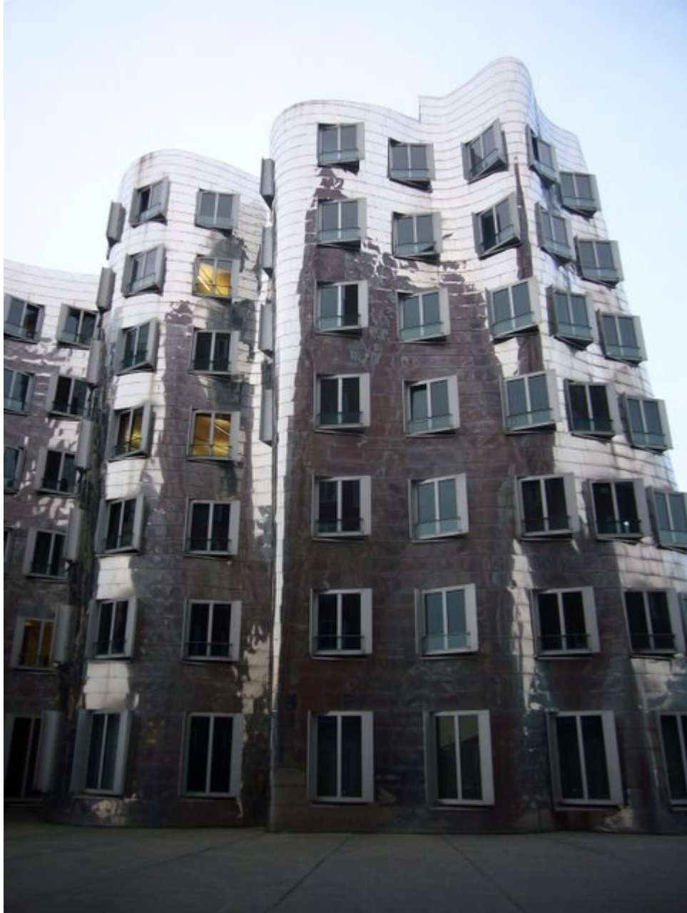
Figure 3.4. Gehry, Dusseldorf Office Building (Source: Kolarevic 2005)
