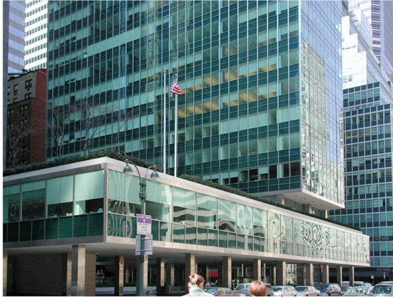
Figure 2.9. Lever Building (Source: Allen 1997)
