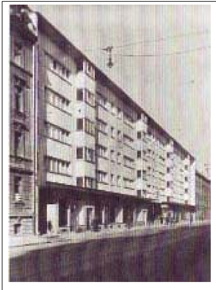
Figure 2.52. The Post Office on Frauenhofer Street by Robert Vorhölzer, Munich, 1929-1931
