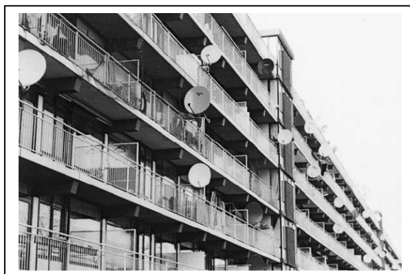
Figure 3. 30. Buildings in Bijlmermeer Project Area (Wassenberg 2004).
