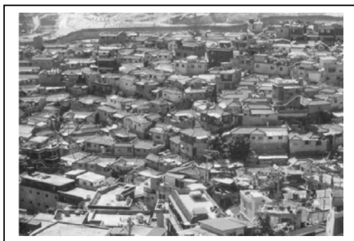
Figure 3. 3. Hapdong Project before clearance (Chang and Jong 2003).
