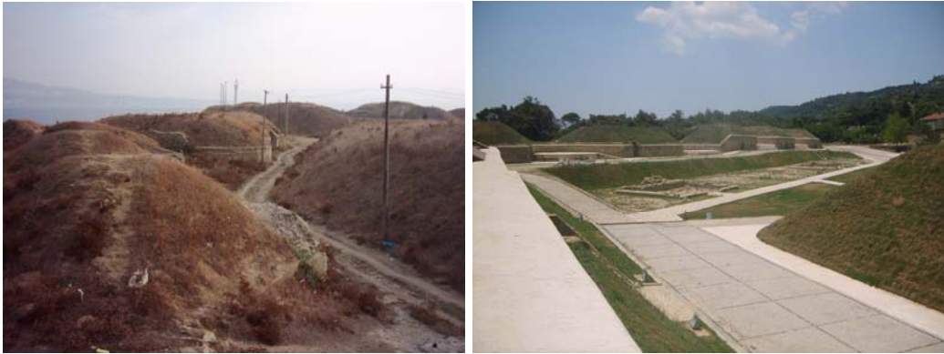
Figure 4.65 Namazgah Rampart, a. before the restoration b. after the restoration (Source: Ahenk Yılmaz archive)
