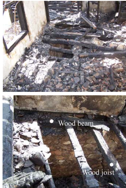
Figure 5.34. Connection detail of ground floor with hımış wall if there is a basement (Şeyh Cami St. No: 32)
