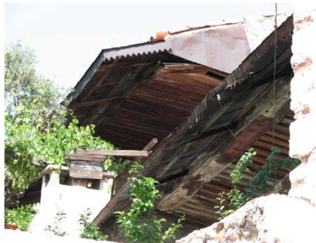
Figure 5.67. Eaves made of galvanized sheets (Topaltı St. No:53).
