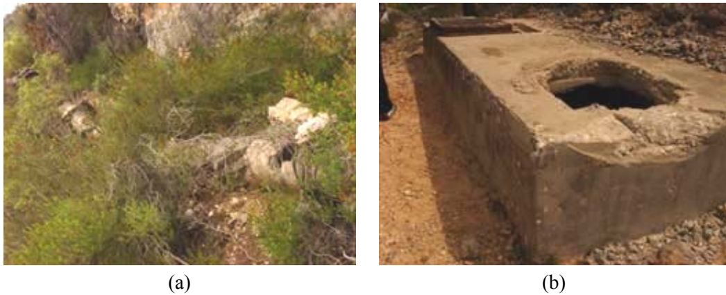
Figure 4.2. a. Pipes of the water supply network, b. water distribution storage
