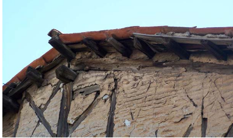
Figure 5.61. Gable wall made of timber-framed totally (Yayla St. No: 13)
