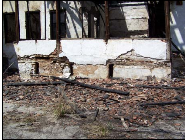
Figure 5.7. Holes left on the exterior façade of the basement for ventilation (Şeyh Cami St.No:32)
