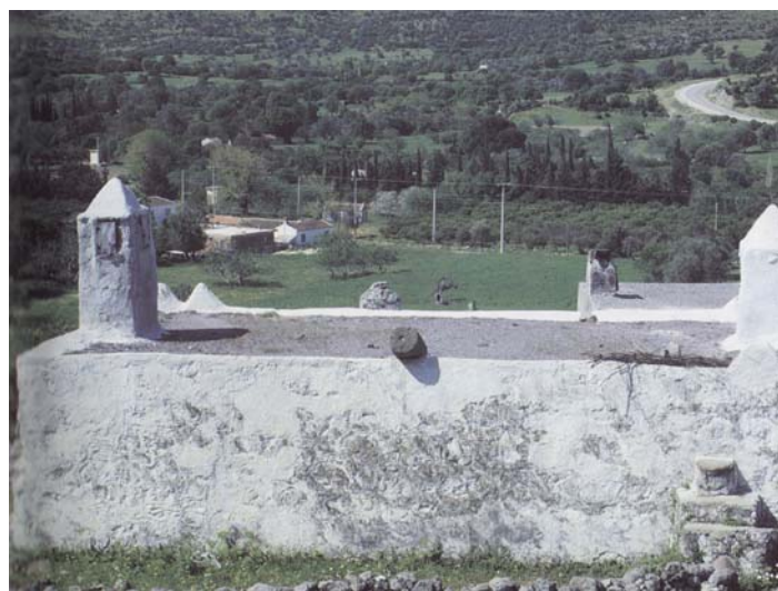
Figure 5.54. Earthen roof in Bodrum – Muğla (Source: Aran 2000)
