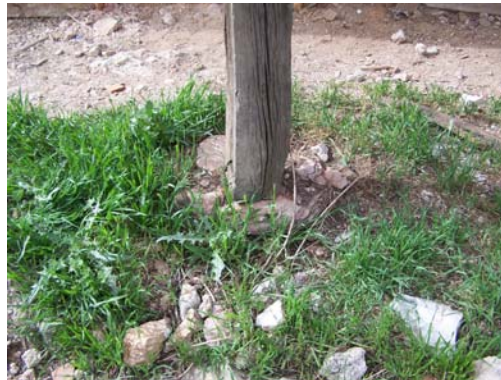
Figure 5.8. Timber post of the sofa placed on a single stone footing (Şahidi St. No: 26)
