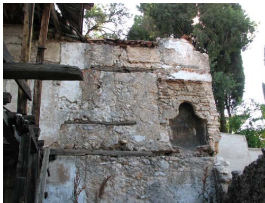
Figure 4.1. The traces on the wall of an additional room in the sofa (Şahidi St. No: 26).
