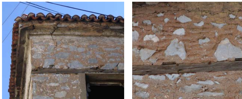
Figure 5.15. Rubble stone wall plastered with ' çivileme ' (Ulucami St. No: 24)
