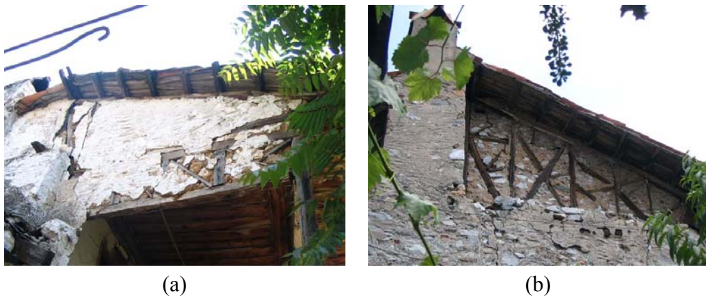
Figure 5.60. Timber-framed gable walls over short sides of sofa; a. Kahveoğlu St. No: 28, b. Süleymanbey St. No: 3
