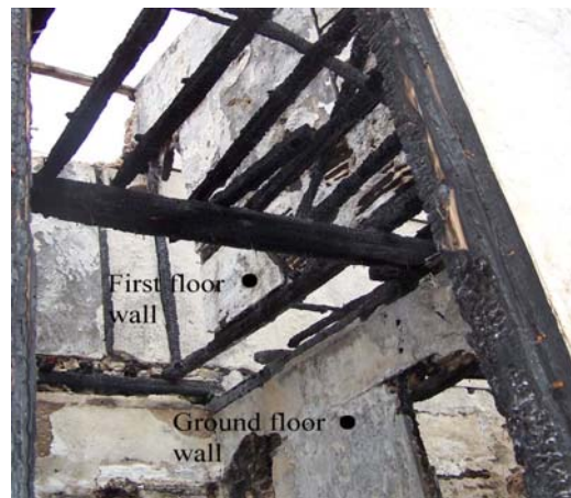
Figure 5.40. Connection detail of timber floor with timber-framed wall (Şeyh Cami St. No: 32)
