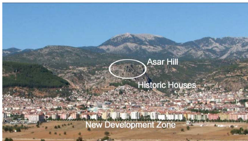
Figure 3.1. General view Muğla from the south
