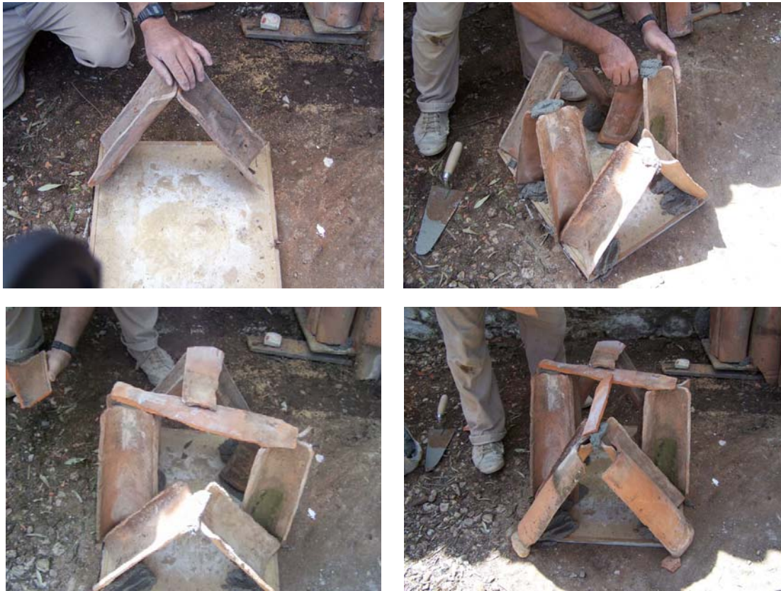
Figure 5.70. The stages of the construction process of chimney cowl of Muğla houses (Source: Ayhan 2008)
