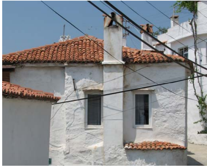
Figure 4.8. Street façade with chimney wall and small windows on its both sides (Şemsiana St. No: 16)
