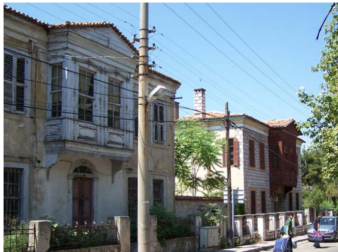
Figure 4.9. Houses which is composed of an entrance door with a cumba above located in the central axis and the windows of the ground and first floors on both sides (Ragıp Bey St. No: 2 and 4)
