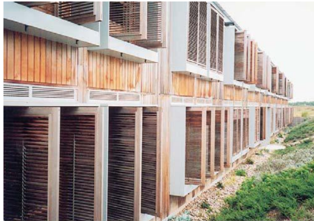
Figure 2.21. External hand-operated louvers to the south east elevation (Source: Phillips 2004)
