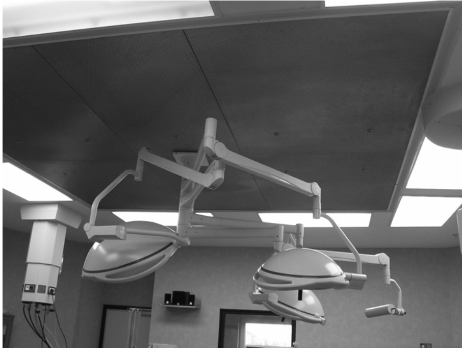
Figure 9.2. Laminar air flow unit installed in the room
