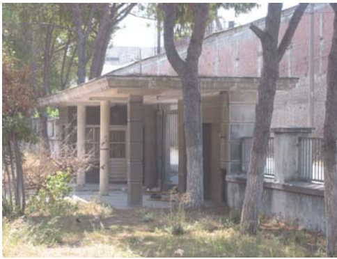
Figure 96. Gate for administrators, İzmir
