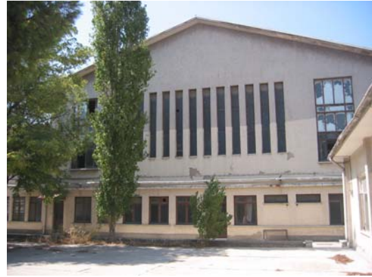
Figure 30. First weaving plant converted to social facilities
