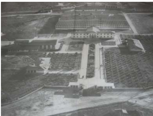
Figure 128. General view, Bergama
