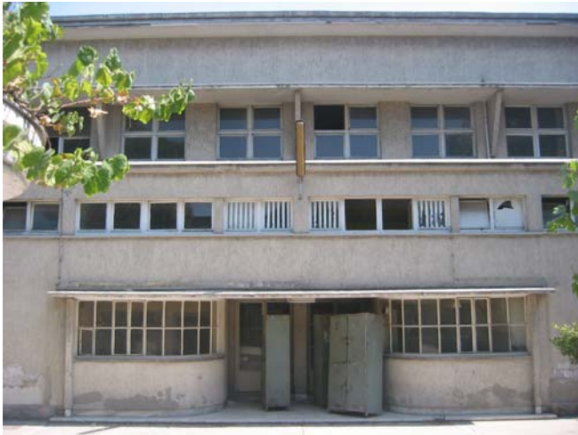
Figure 35. Entrance for labourers (Source: Courtesy of Deniz Güner)
