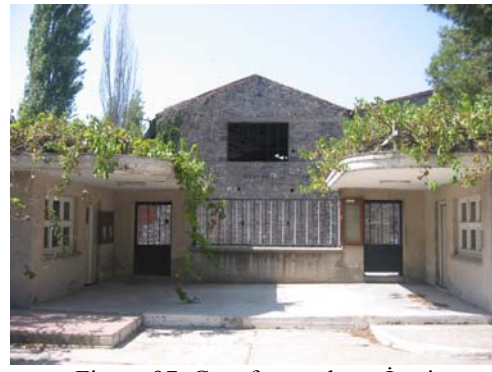
Figure 97. Gate for workers, İzmir
