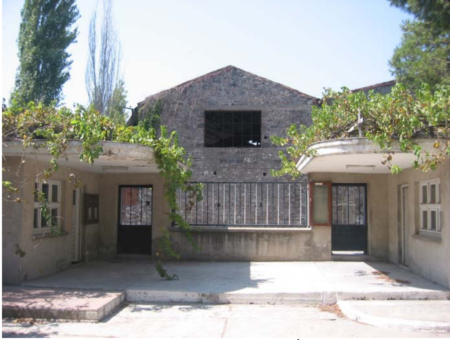
Figure 123. Gate for workers, İzmir
