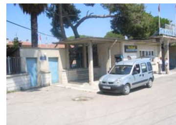
Figure 120. Gate for workers, Manisa
