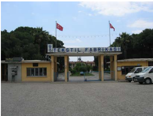
Figure 49. Main gate of the Campus
