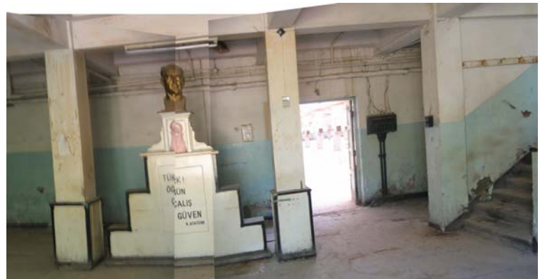
Figure 19. Production hall entrance for workers
