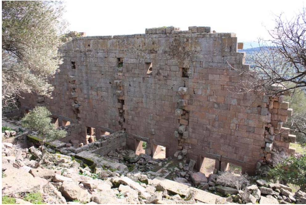
Figure 9. Collapsed parts inside of the building
