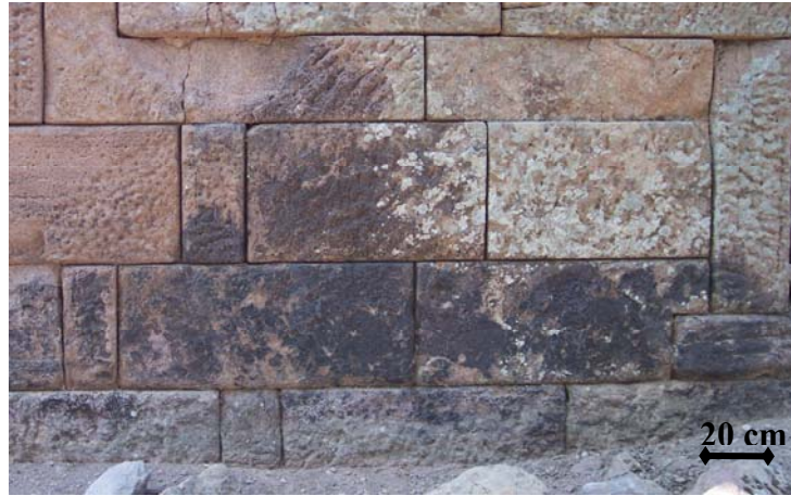
Figure 28. Black crust observed on the stone surfaces of Agora
