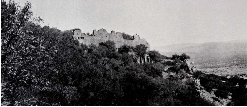
Figure 11. Southeast wall of Agora in 1886 (Source: Bohn and Schuchhardt 1889)
