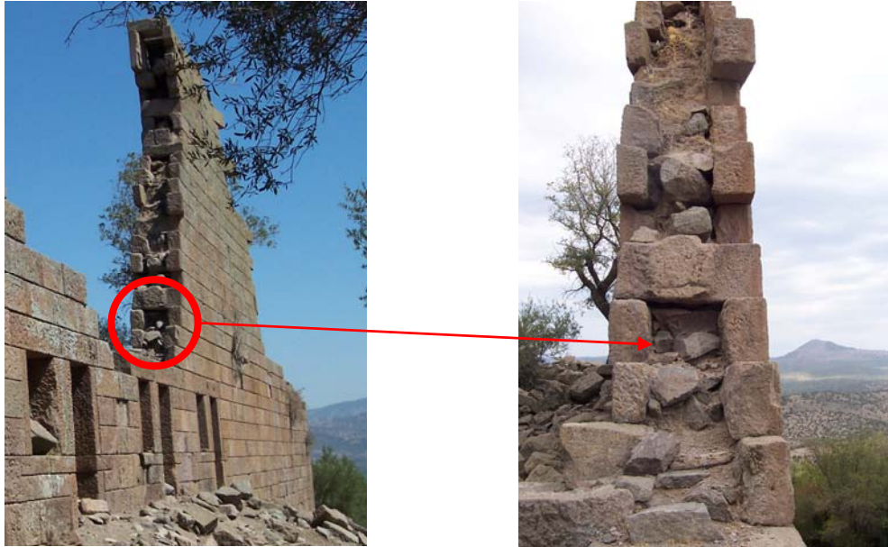
Figure 48. Rubble core, showing where infill materials were collected (A.S)
