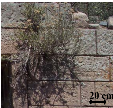
Figure 30. Higher plants observed on some parts of Southeast facade of Agora
