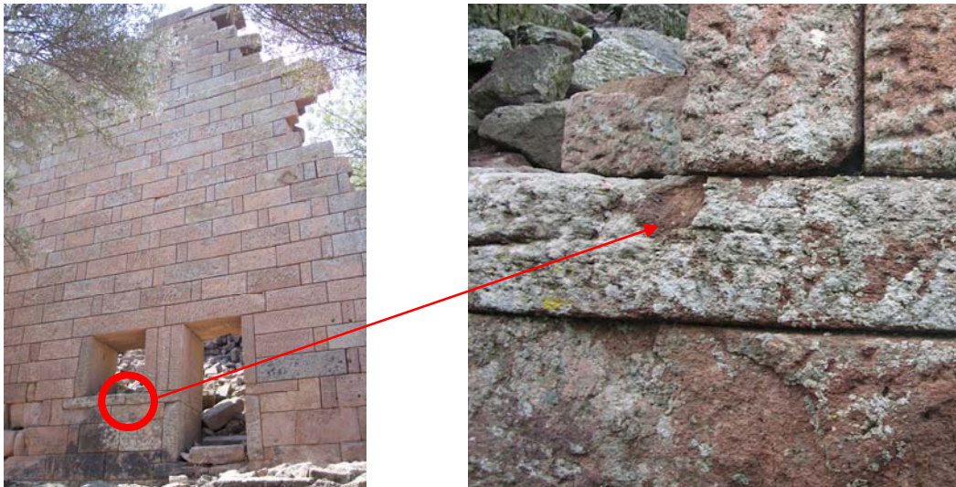
Figure 47. Southeast facade of the wall, showing where the andesite samples were collected (A.St.4)
