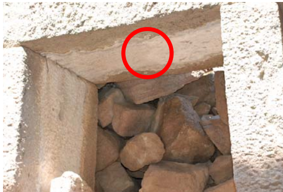
Figure 49. Lintel of 7 th chamber showing where samples of efflorescence were collected (A.Eff.1)
