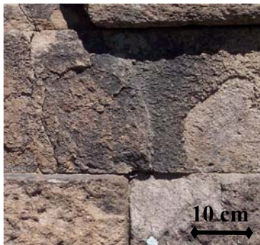
Figure 36. Detachment of black crust observed on the stone surfaces of Agora
