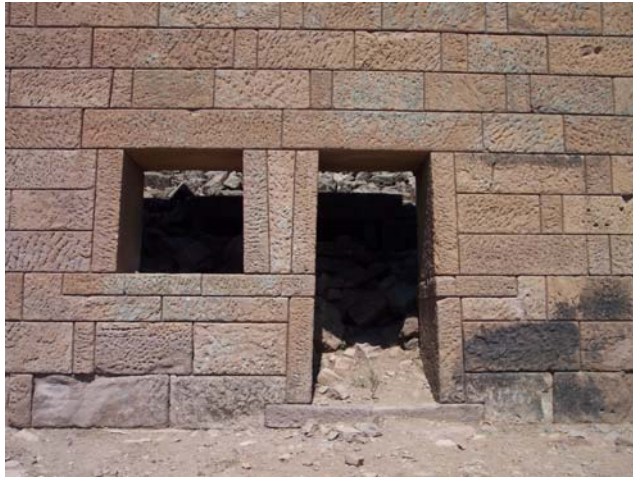
Figure 6. Entrance door and window openings of the 6 th chamber
