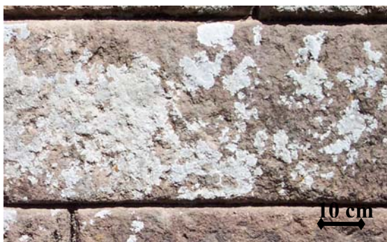
Figure 26. Microbiological colonization observed on the stone surfaces of Agora
