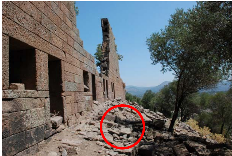
Figure 45. Collapsed building stones, showing where the andesite samples were collected (A.St.1 and A.St.2)
