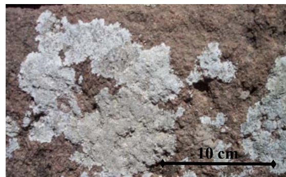
Figure 27. Microbiological colonization observed on the stone surfaces of Agora
