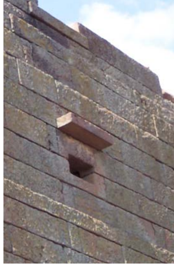
Figure 8. Sun-breakers on the facade of the third floor
