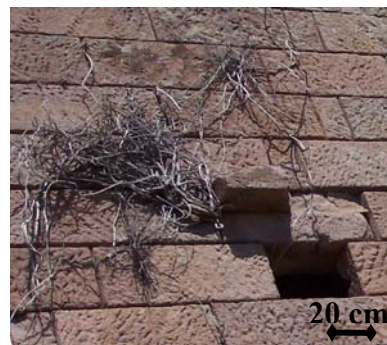
Figure 31. Higher plants observed on some parts of Southeast facade of Agora
